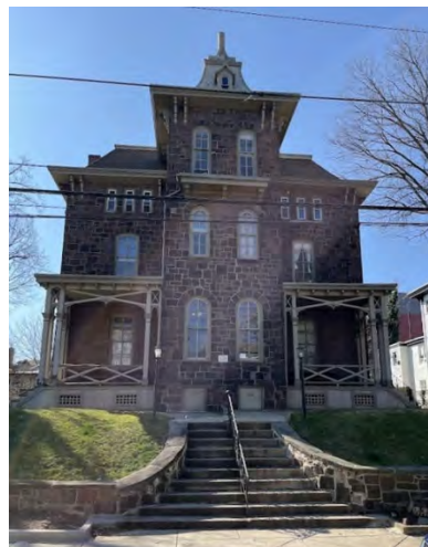
Figure 12. 4004 and 4006 Pine Street, view to southwest.
