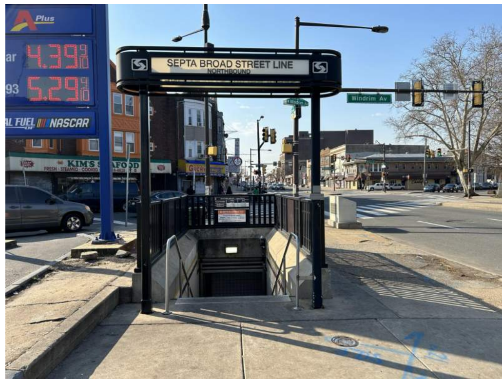
SOUTHEAST ENTRANCE (NORTHBOUND)
