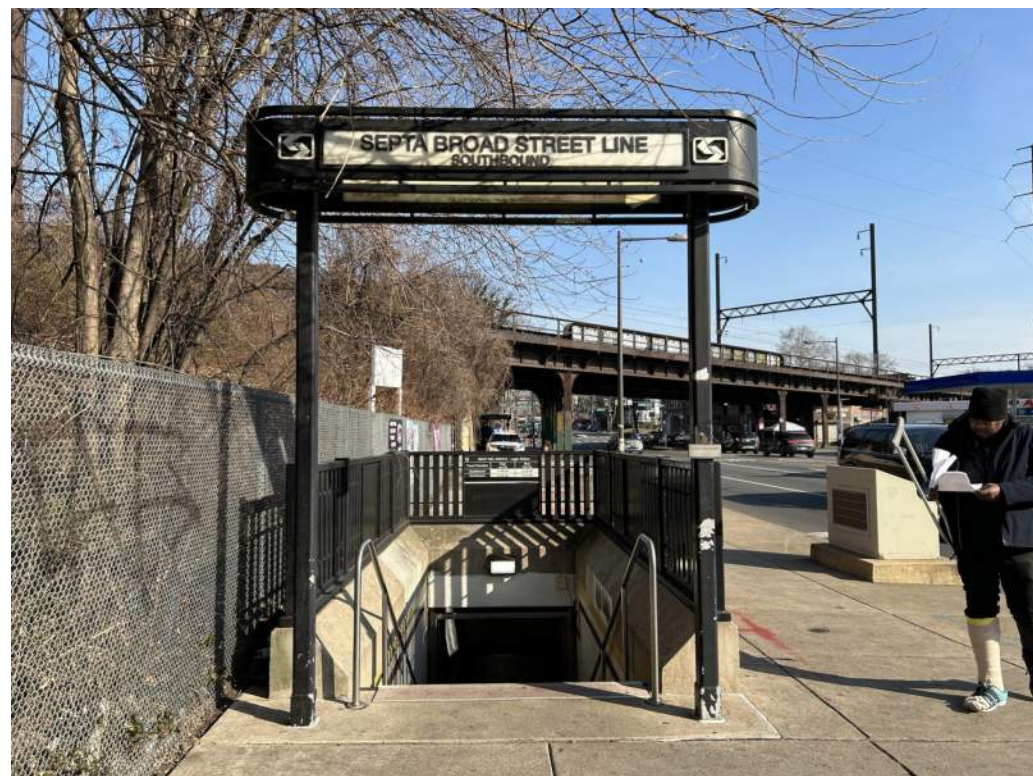
SOUTHWEST ENTRANCE (SOUTHBOUND)
