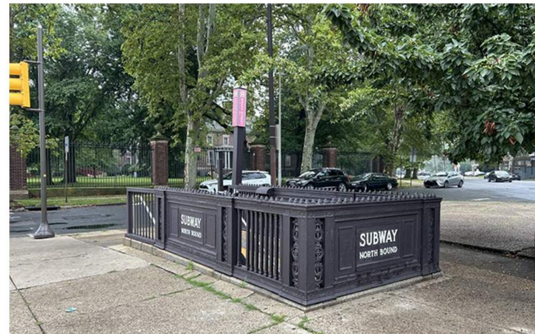
NORTHEAST STATION ENTRANCE
