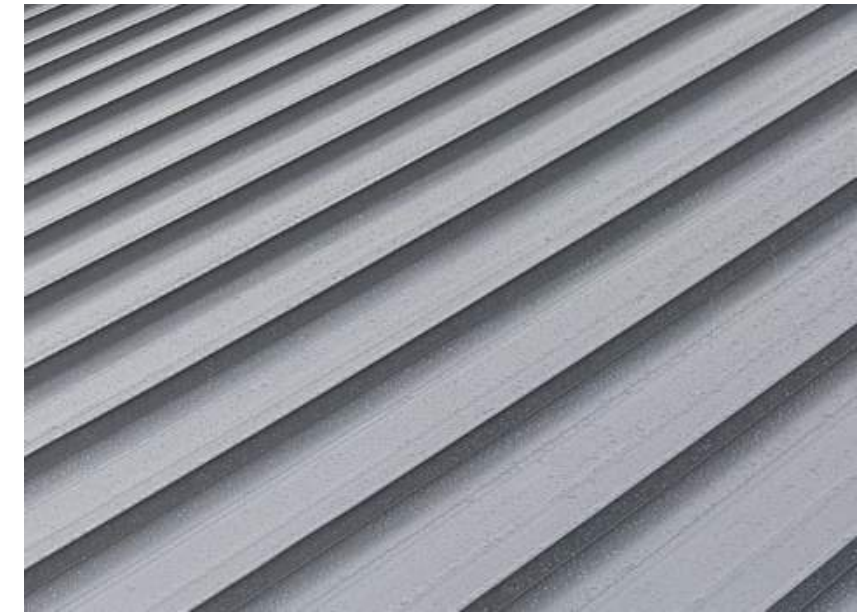
STANDING SEAM ROOF
