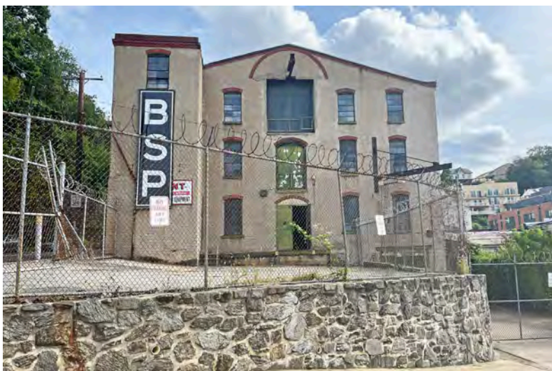
Photo 1: West elevation, looking east.
