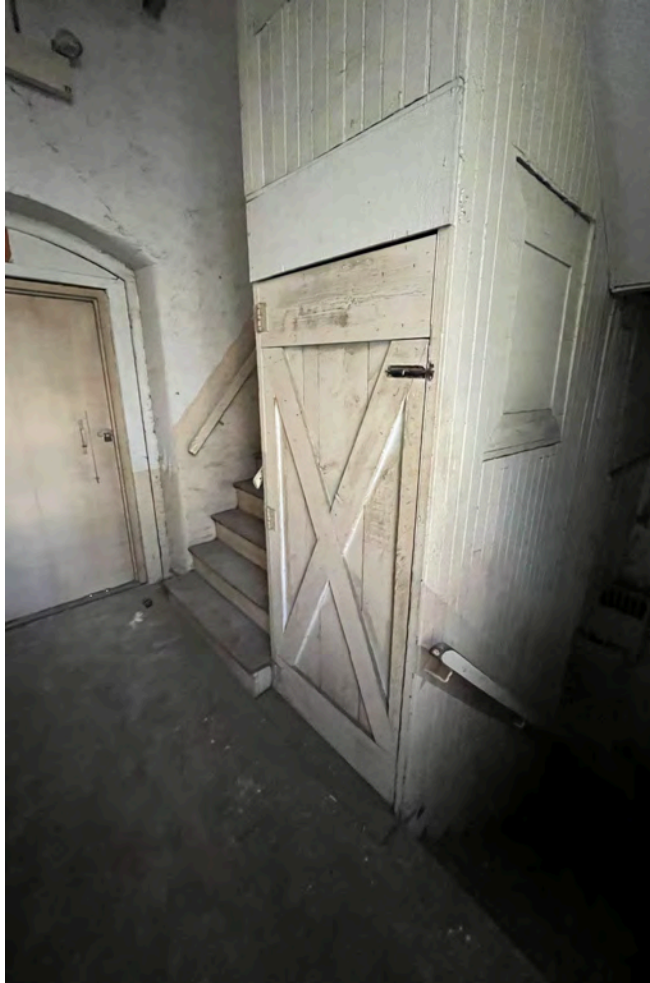
Photo 13: Stair tower interior, looking southwest on the 1st floor.
