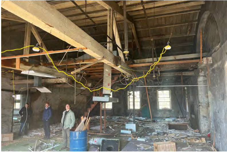
Photo 11: 3rd floor, looking north.
