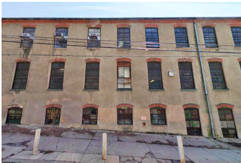
Photo 3: Central portion of the north elevation, looking south.
