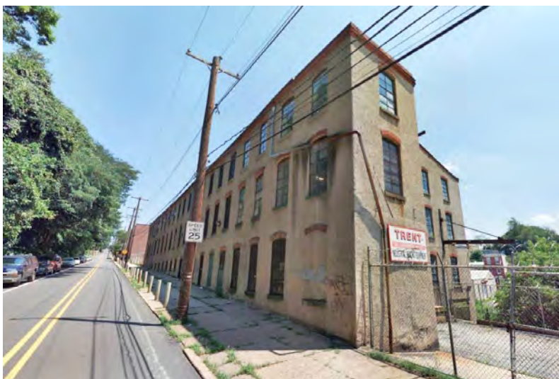
Photo 2: North and west elevations, looking southeast.
