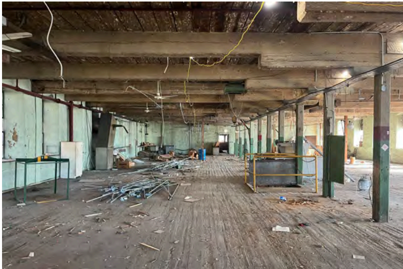
Photo 10: 2nd story, looking east.
