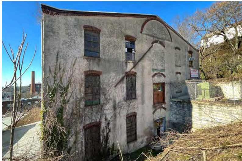
Photo 5: East elevation, looking northwest.
