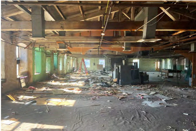
Photo 12: 3rd floor, looking west.
