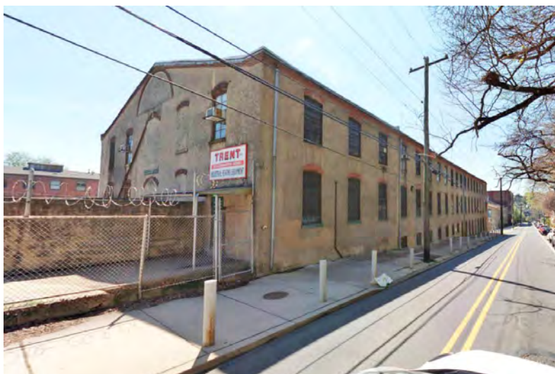
Photo 4: East and north elevations, looking southwest.
