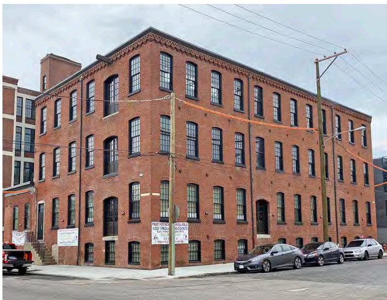
Figure 9: The Franklin Carpet Mill at 2139-45 E. Huntingdon Street in Philadelphia, built between 1879 and 1892. This mill is typical of those built in and around Kensington during the late nineteenth century. Photo from Powers & Company.
