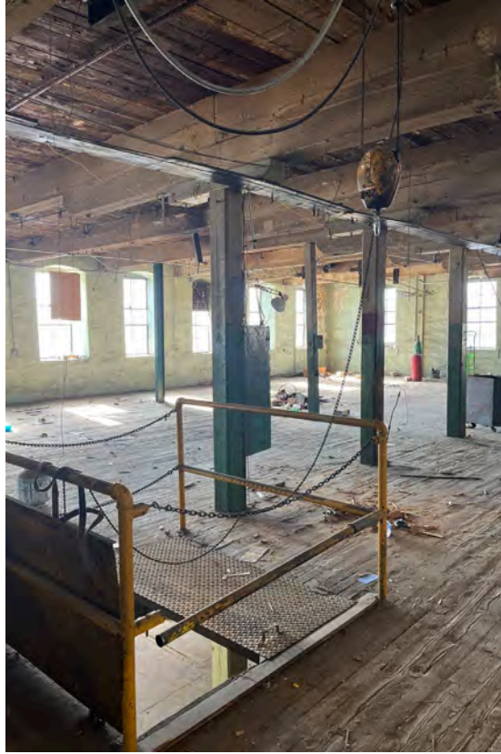
Photo 9: 1st floor, looking southwest.
