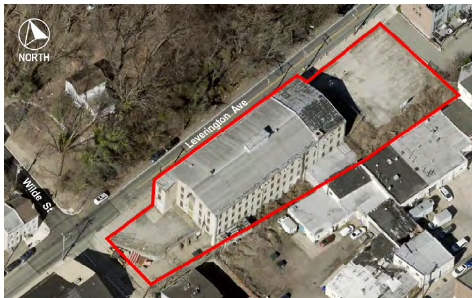
Figure 1: Aerial view showing the Keystone Mill in 2023 (Pictometry).
