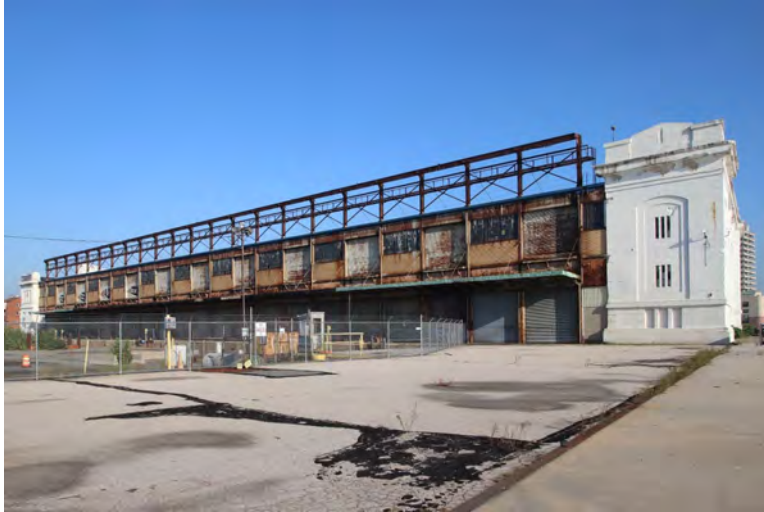
Photo 7: South elevation of Pier 38, looking northwest.
