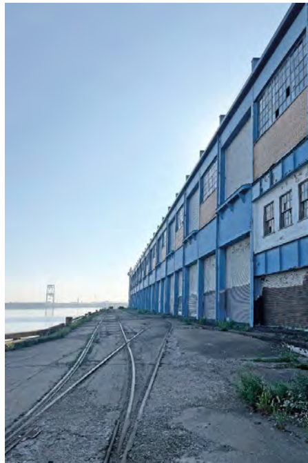
Photo 6: North elevation of Pier 38, looking east.
