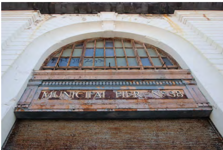
Photo 3: West elevation of Pier 38, detail of the center bay, looking east.
