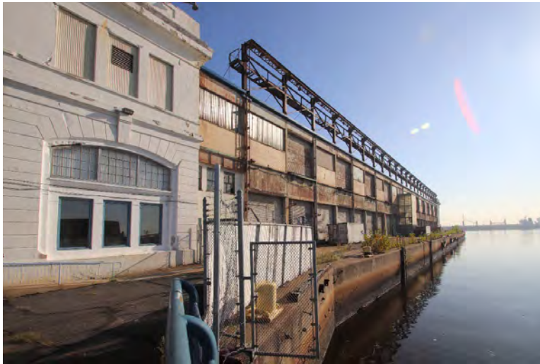
Photo 9: South elevation of Pier 40, looking northeast.
