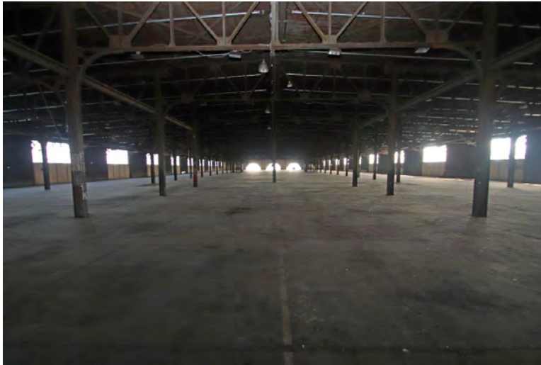
Photo 14: Second story of Pier 38, looking east.
