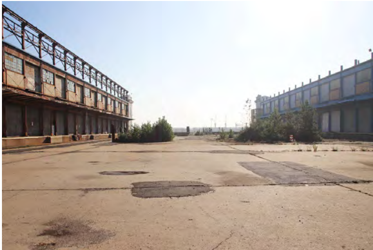
Photo 10: The area between the two piers, looking east toward the river.
