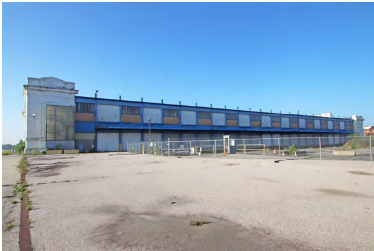
Photo 8: North elevation of Pier 40, looking southwest.
