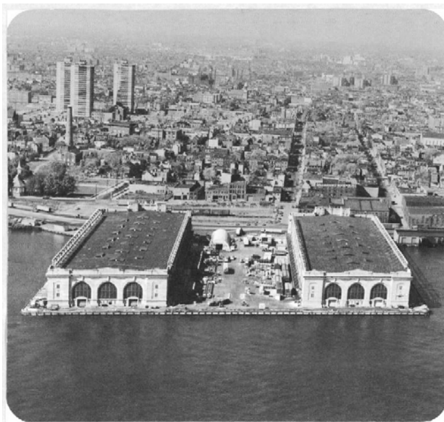
Figure 20: Outshore aerial view of the Southwark Municipal Piers in the 1970s, showing the concrete deck that was built between the buildings in 1957-58 (Port of Philadelphia).
