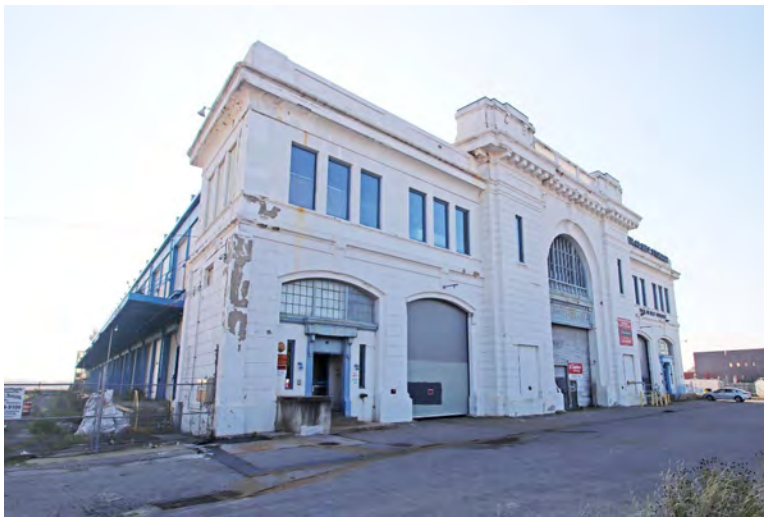
Photo 2: West elevation of Pier 40, looking southeast.
