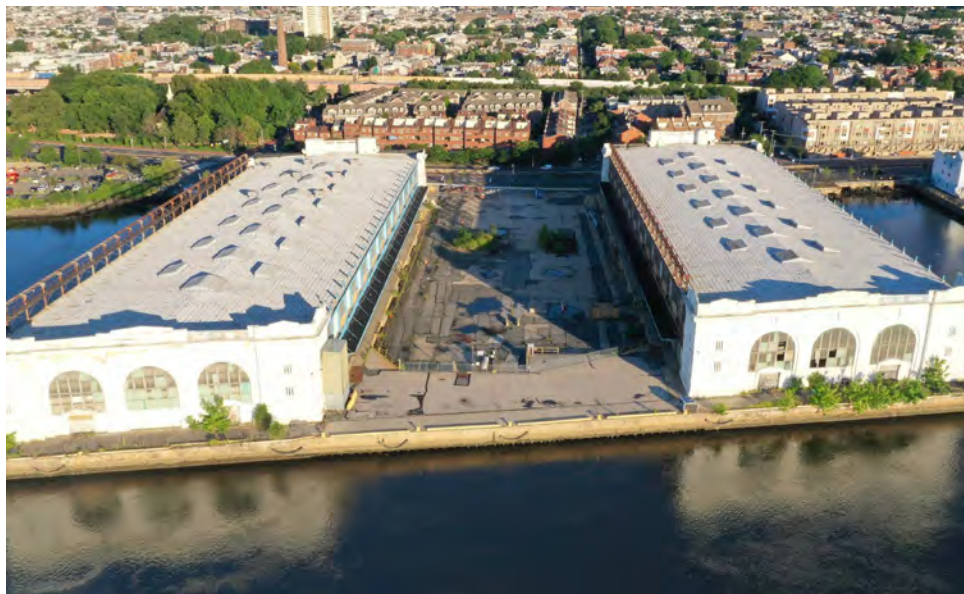
Figure 1: Aerial view of the Southwark Municipal Piers in 2022, looking west (Binswanger). Pier 38 is on the right and Pier 40 is on the left.
