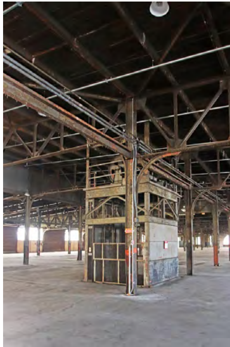
Photo 16: Freight elevator on the second story of Pier 38, looking southwest.
