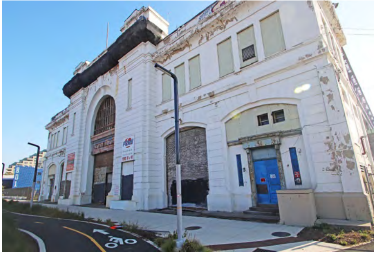
Photo 1: West elevation of Pier 38, looking northeast.
