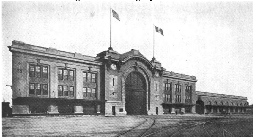
Figure 15: Inshore view of Pier 78, South Wharves, one of the Moyamensing Piers, designed by the Department of Wharves and built 1919-20. Extant (from the Annual Report of the Department of Wharves, Docks and Ferries , 1918). Pier 84, completed in 1926, is similar in appearance. Piers 80 and 82, which were not built until 1952 and 1941, respectively, were much more utilitarian in their architectural treatment.
