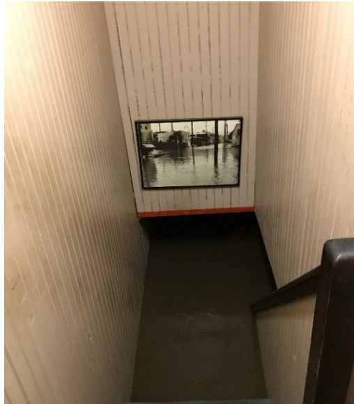
Figure 6: Flood waters entering existing office stairwell.
