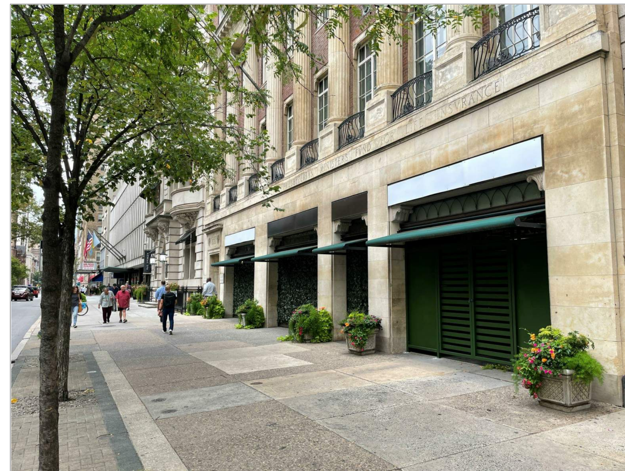
VIEW DOWN THE BLOCK LOOKING WEST- EXISTING AWNINGS PROJECT 4'-1" FROM STONE FACADE
