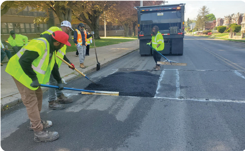
A resurfacing crew works on a Philadelphia street.
