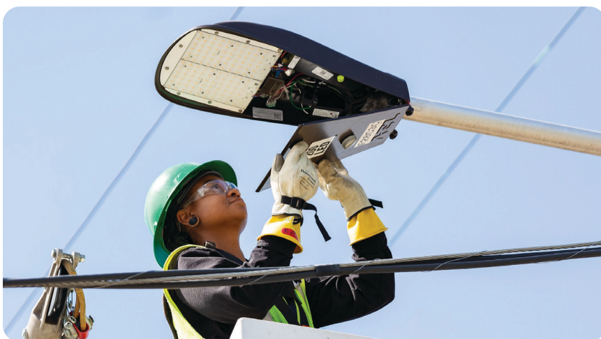
A Streets Department employee installs an LED streetlight.
