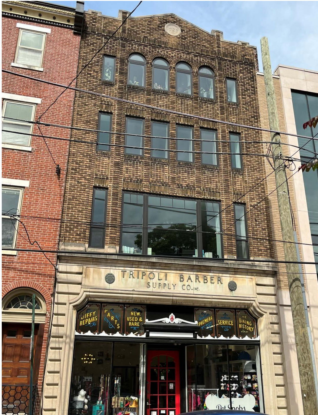
Figure 5. Front facade of 606 S. 9th Street, November 2023.
