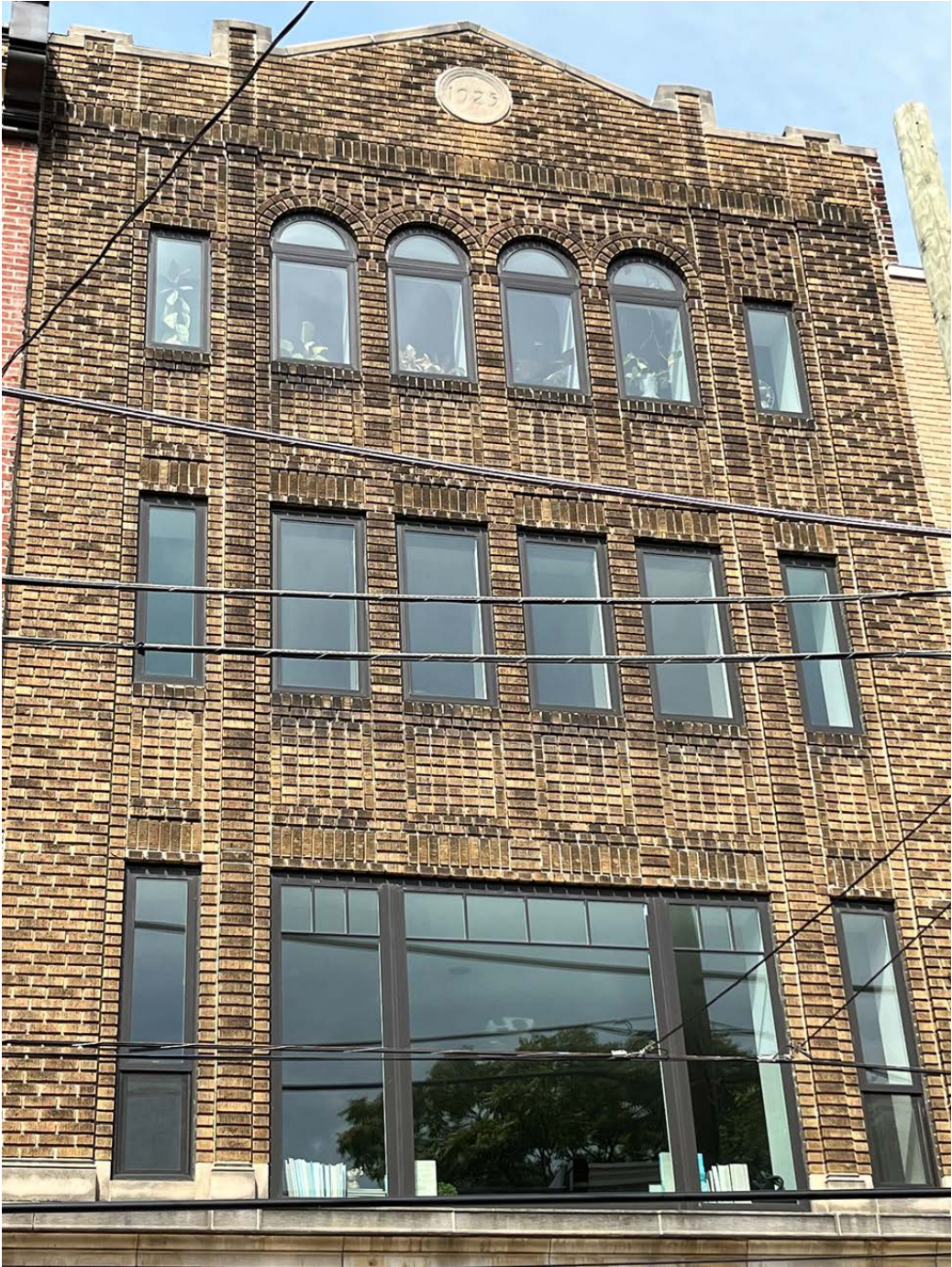
Figure 6. Floors two through four of primary façade, November 2023.
