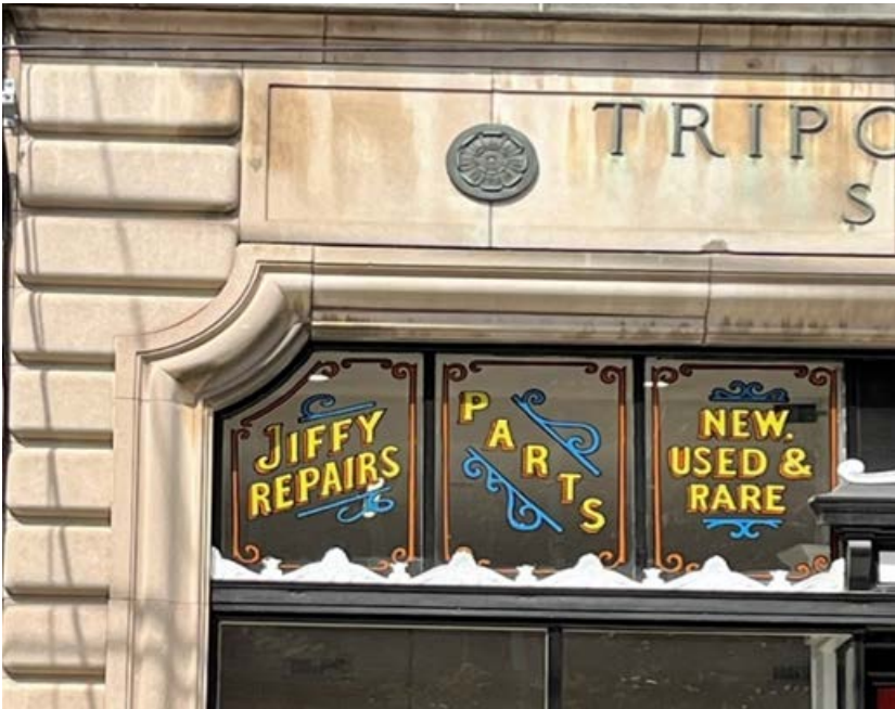
Figure 8. 606 S. 9th St. storefront detail, November 2023.
