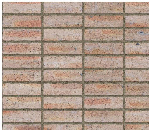
BRICK VENEER B (ALTERNATE 1) STACKED BOND COLOR: BEIGE MORTAR: KLM KEYSTONE
