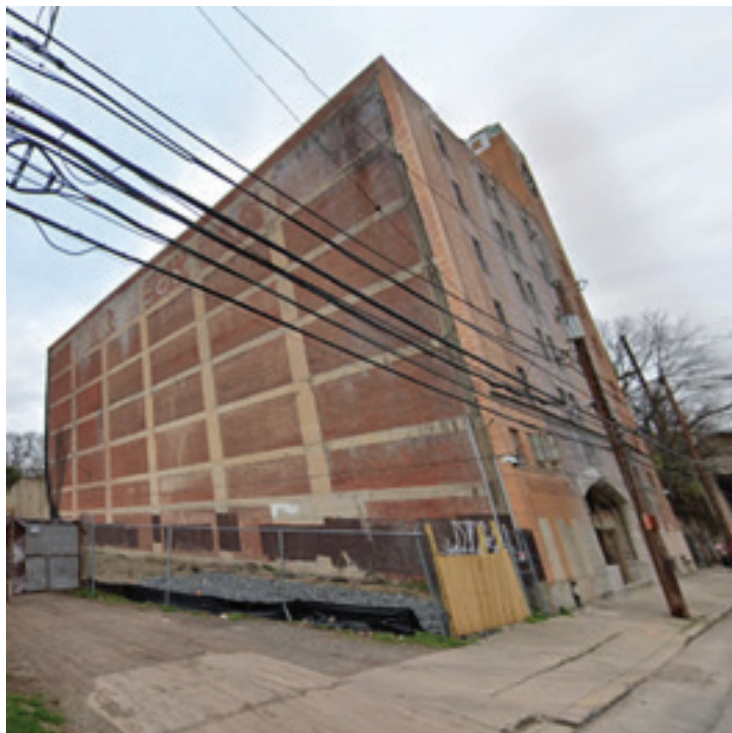
BUILDING B 231 CHURCH LN. (7 STORIES)
