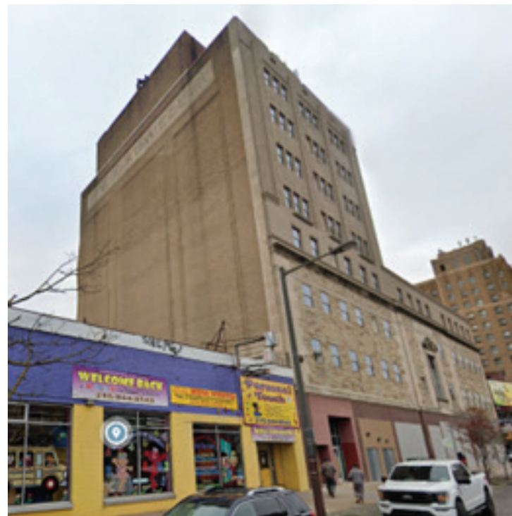
BUILDING D 40 E. CHELTEN AVE. (8 STORIES)
