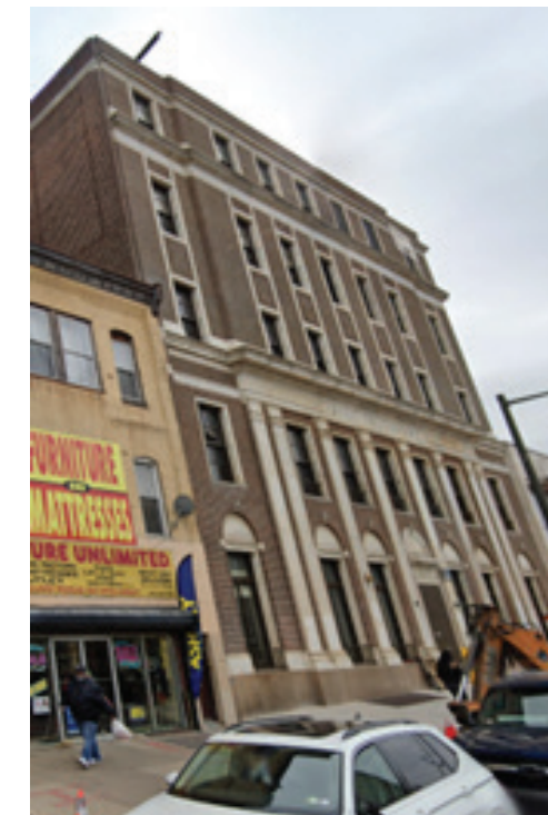
BUILDING F 26-34 W. CHELTEN AVE. (5 STORIES)
