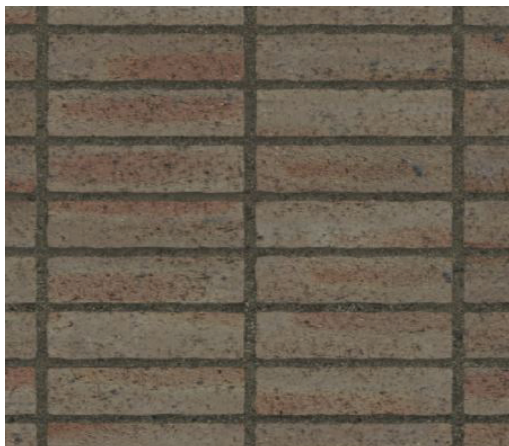
BRICK VENEER B STACKED BOND COLOR: TAUPE MORTAR: KLM KEYSTONE
