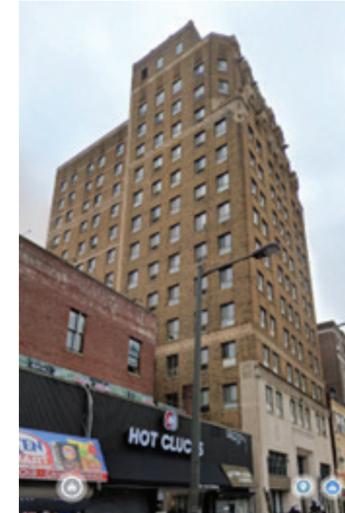
BUILDING E 18 W. CHELTEN AVE. (14 STORIES)
