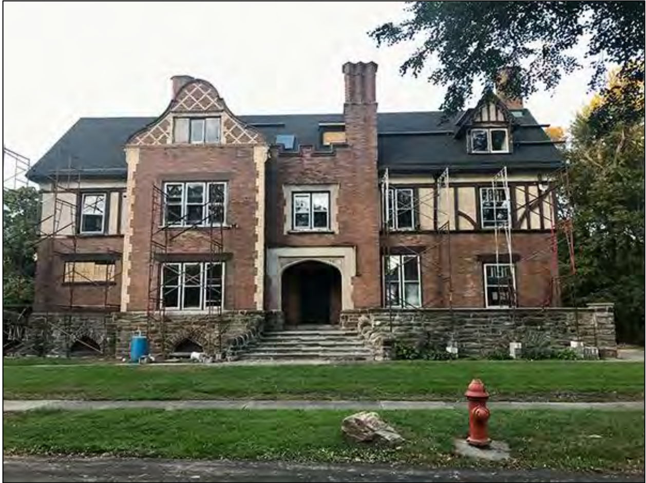
Fig. 3. West and primary elevation of Overleigh, October 13, 2023.
