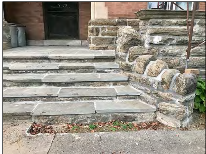
Figs. 20 & 21. Left, a typical window with three gothic-arched transoms infilled with leaded, diamond coming within a wood sash. Right, the front steps after modification in early 2023 to match the north cheek wall, interrupting Pearson's delineation between public & private sides. October 13, 2023.
