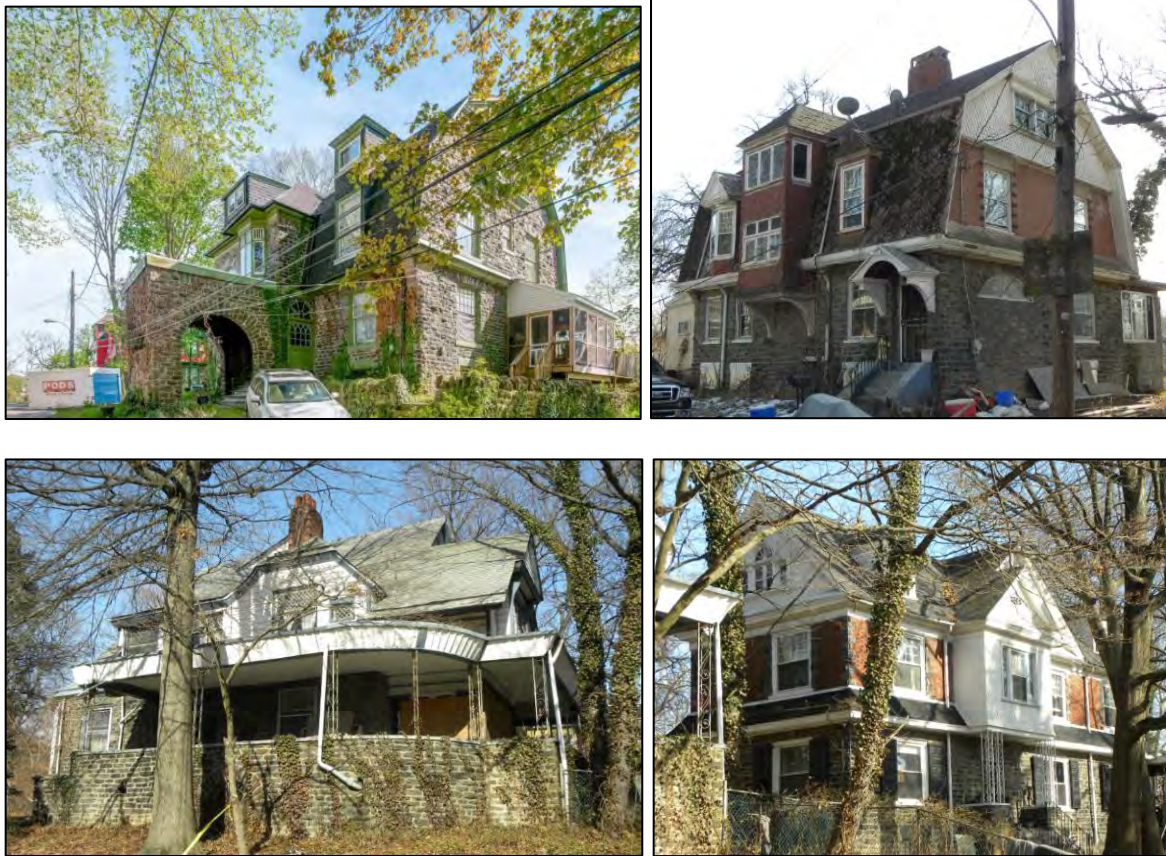
Figs. 38, 39, 40, and 41. The four Pearson-designed houses for John T. Roberts on Wingohocking Heights: Source: Aaron Wunsch, 2016.
