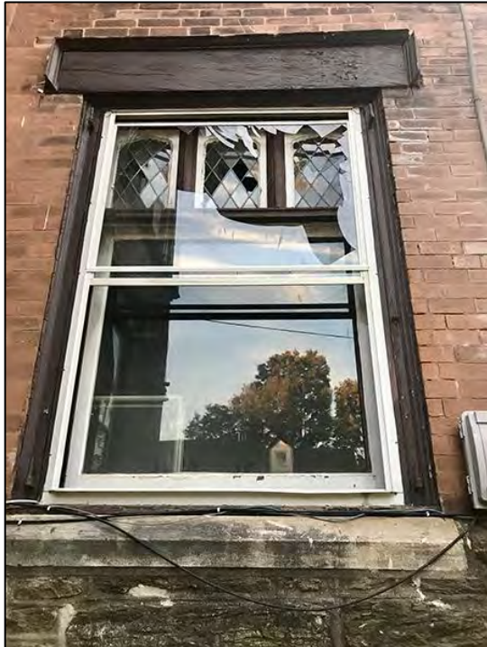
Figs. 20 & 21. Left, a typical window with three gothic-arched transoms infilled with leaded, diamond coming within a wood sash. Right, the front steps after modification in early 2023 to match the north cheek wall, interrupting Pearson's delineation between public & private sides. October 13, 2023.
