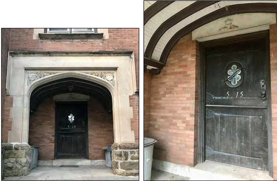
Figs. 5 & 6. Left, the front entry portal framed in honed limestone with Tudoresque flourishes and heraldic shields. Right, the original front door in the Dutch style with decorative ironwork. Both photos, October 13, 2023.
