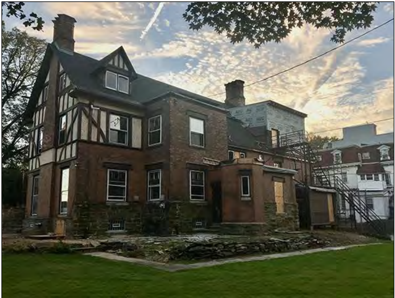
Fig. 12. The southeast corner of Overleigh, looking at the rear elevation. October 13, 2023.
