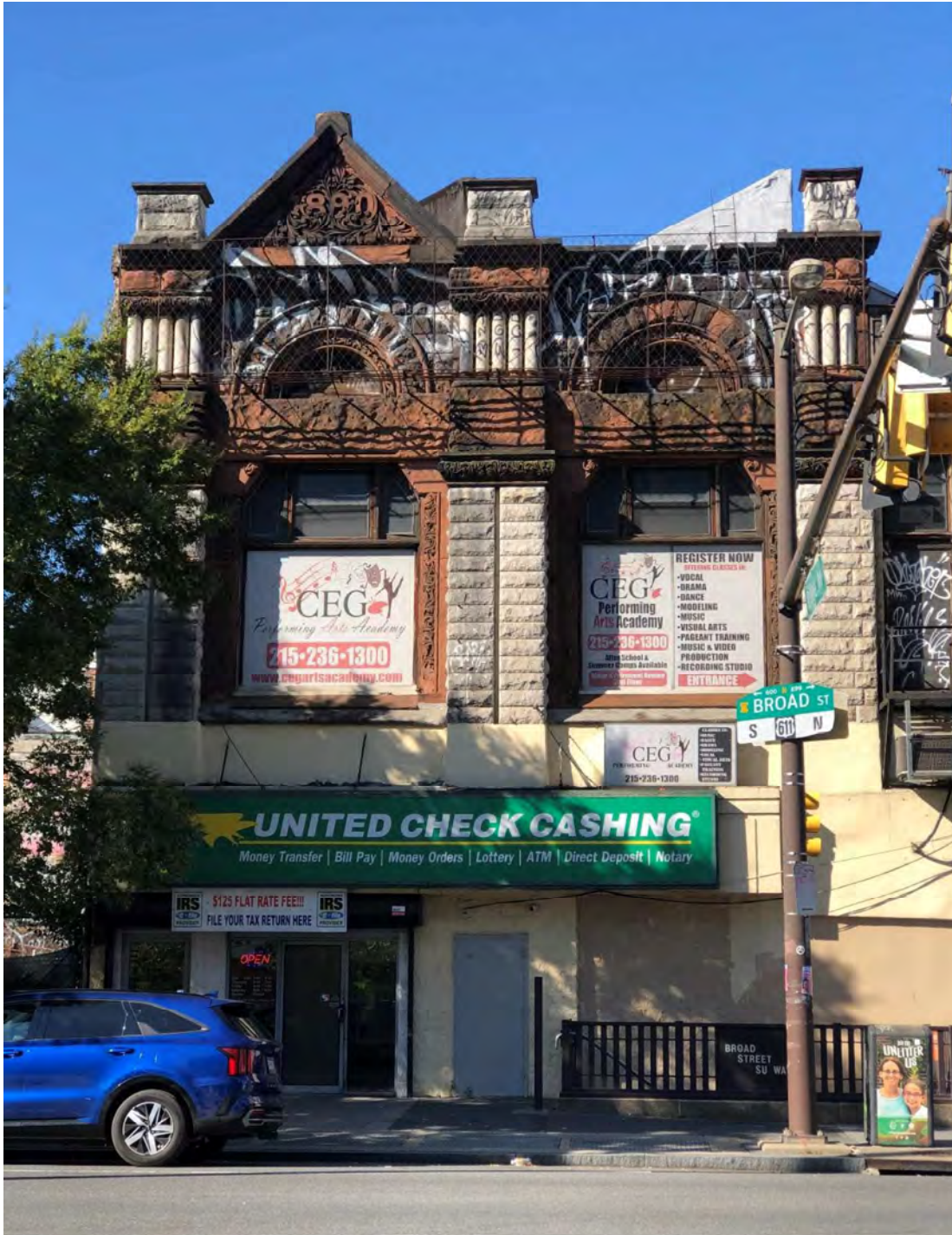
Figure 3. Front façade of 684-86 N Broad Street. A contemporary storefront and subway entrance are at the first floor. The building's second and third floors retain their original material and details. Between 2022 and 2023, the third floor was vandalized with graffiti, covering up the polychrome masonry. Image source: PHC staff, 2023.
