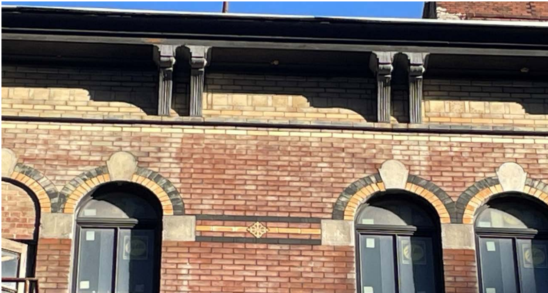
Figure 39: Detail showing the fourth-floor ornament as well as the cornice, which features a band of tiles as well as several courses of colored bricks. This elevation was previously painted, obscuring some of the flourishes.
