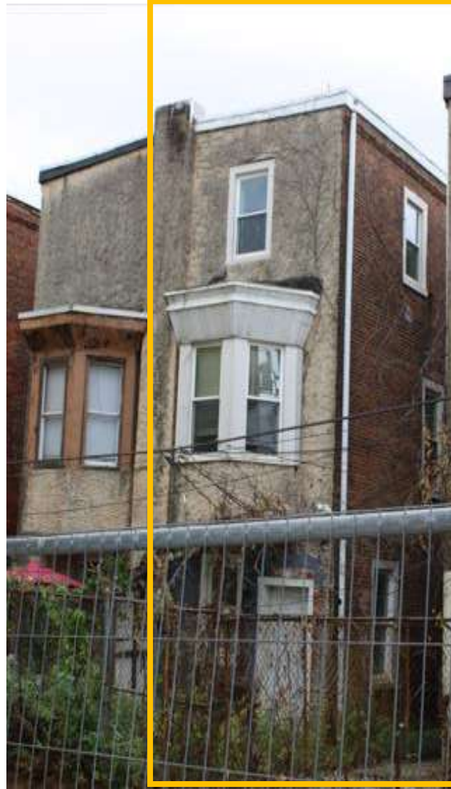
Figure 6. Rear elevation. Credit: Laurie Wexler
