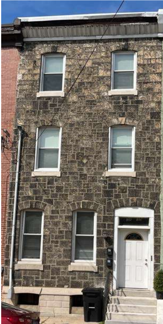
Figure 5. Façade. Credit: Laurie Wexler
