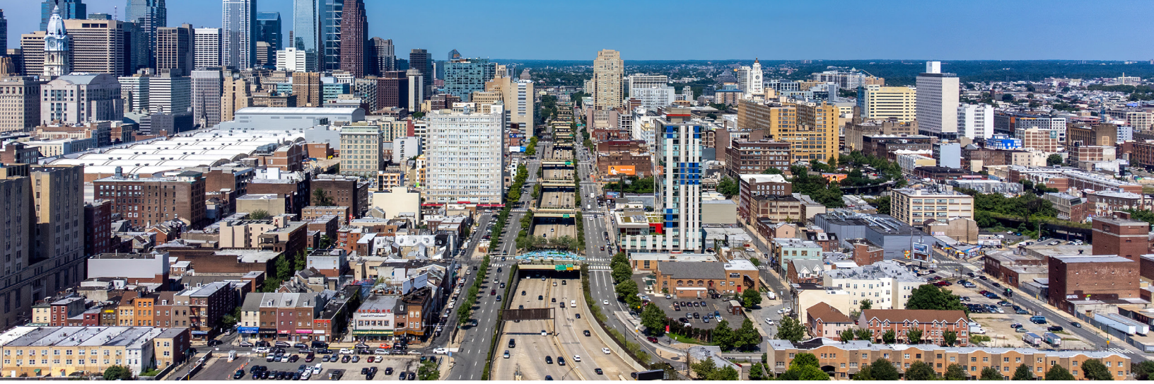
Image: The Chinatown Stitch received a $1.8 M Reconnecting Communities grant through BIL. The project will study a cap over the expressway and Vine Street improvements.
