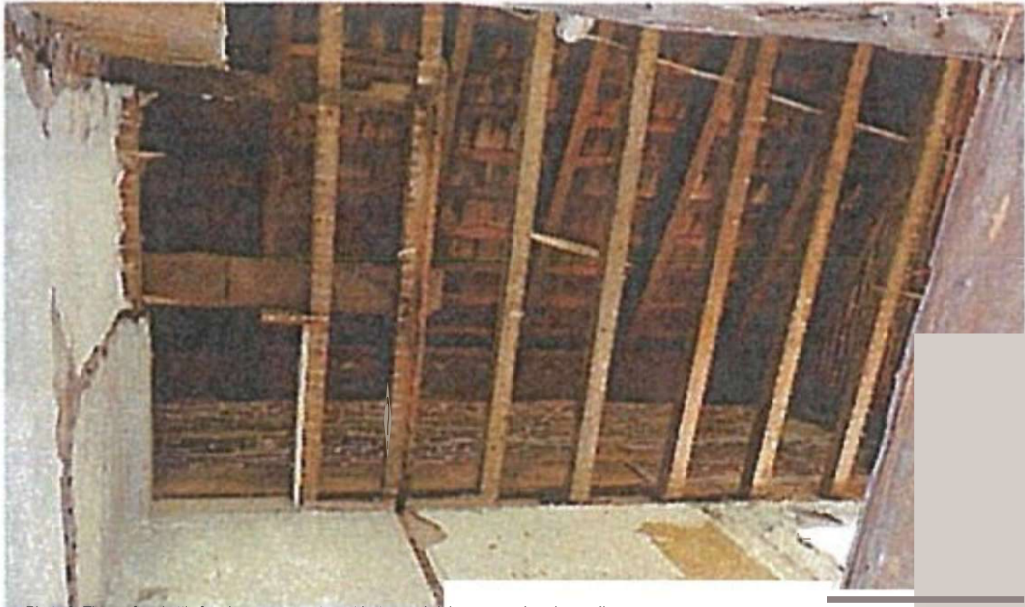
Photo 2: The roof and attic framing spans east-west between brick masonry bearing walls.
