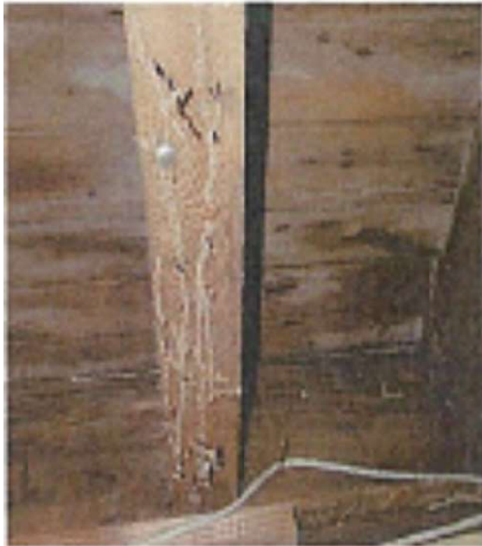
Photo3: There is evidence of insect damage on the underside of the first floor framing.
