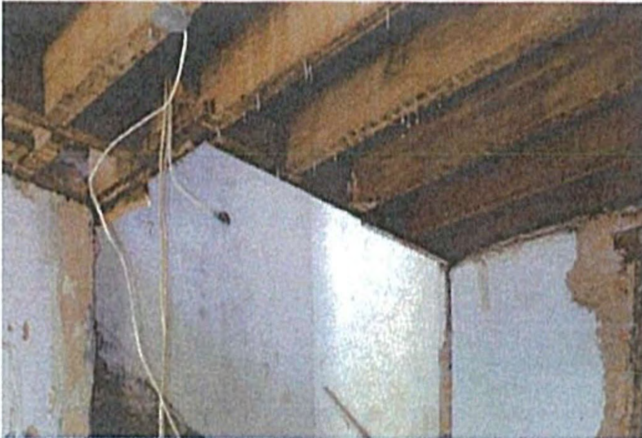
Photo 1: The stair header and the fireplace header are supported by a single member trimmer joist.
