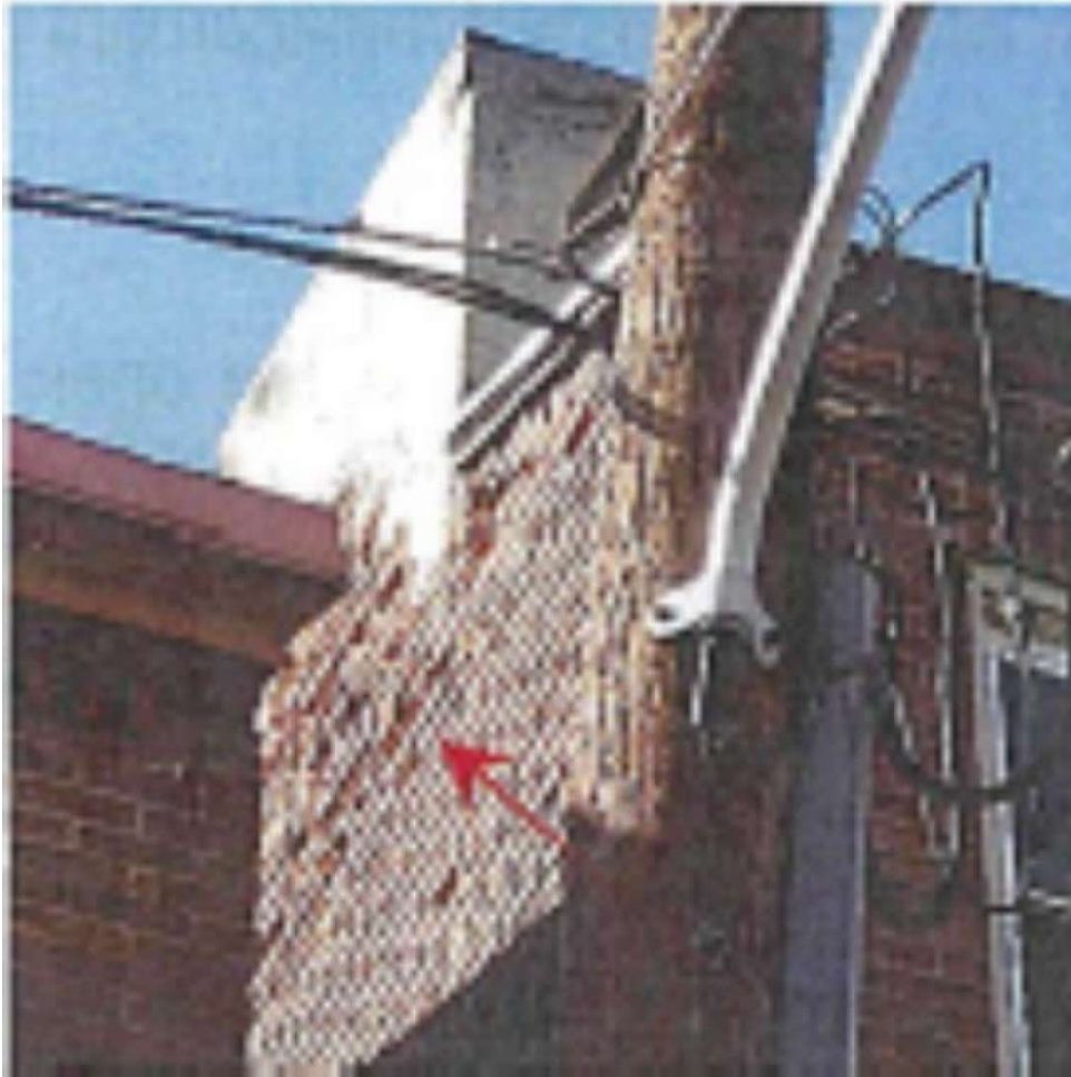
Photo 9: At the top of the south elevation, the wall exhibits open mortar joints and deteriorated brick.
