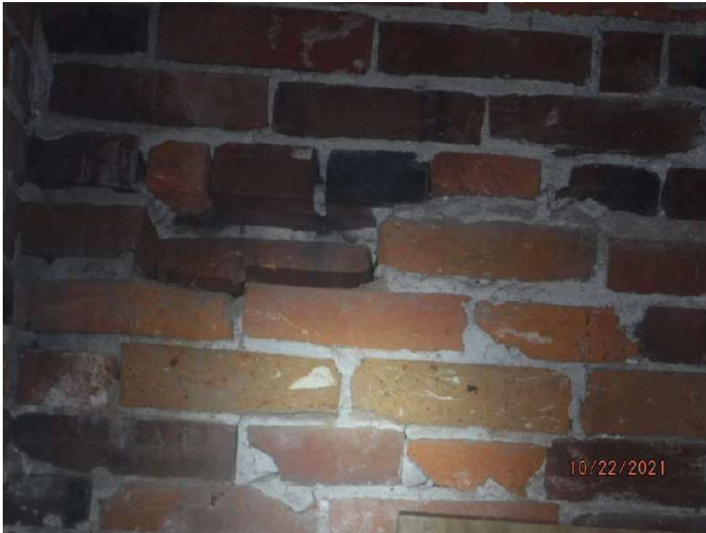
INTERIOR DETERIORATED BRICK
