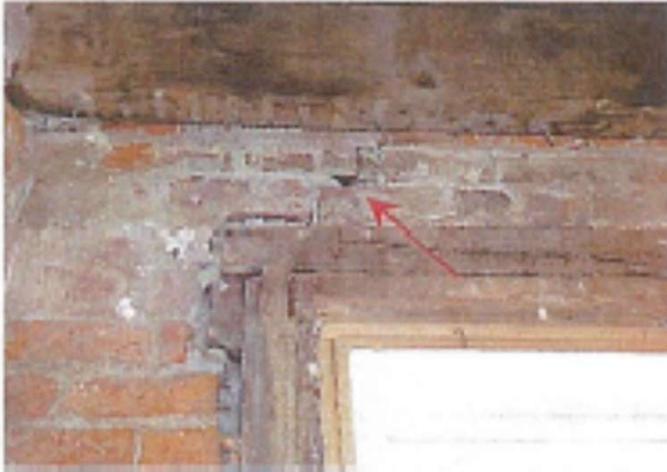
Photo 7: Some of the cracks on the east elevation extend through the full thickness of the wall.
