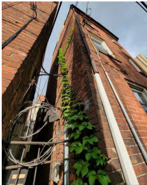
Image No. 7- Loose masonry/ masonry voids at the exterior wall
