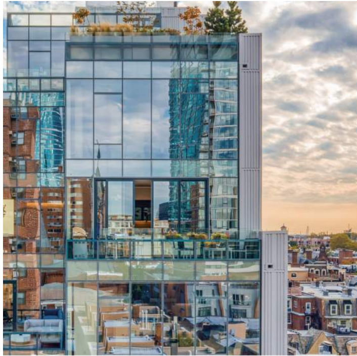
1 2 Window Wall System with Spandrel
