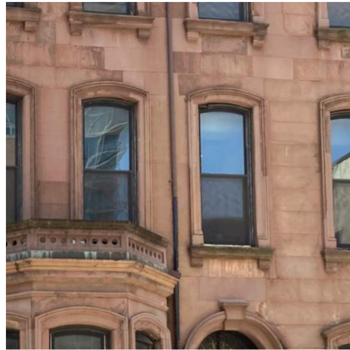
6 Existing Masonry to be Restored
