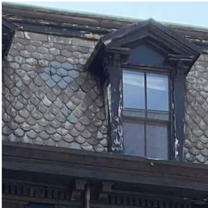
5 Existing Slate Shingles to be Restored
