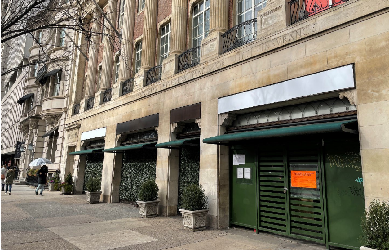
Figure 1. Existing conditions at 1805-09 Walnut Street, January 2024.
