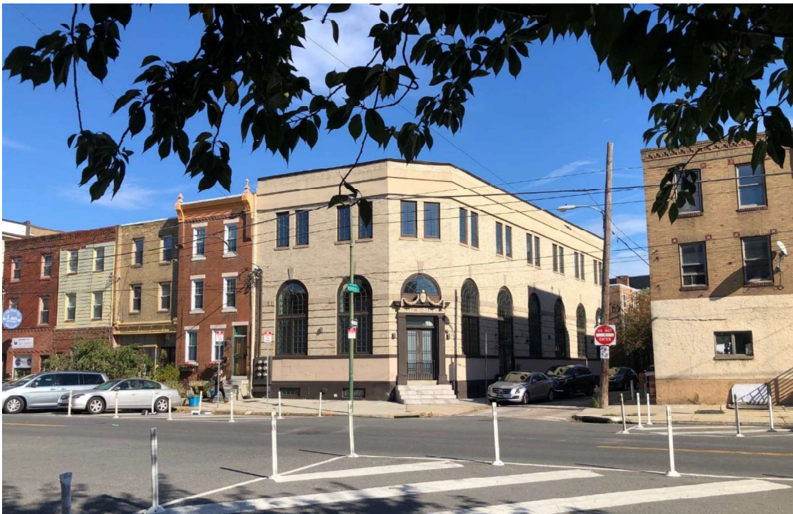
Figure 3: View of S. 11 th Street and Montrose Street facades.
