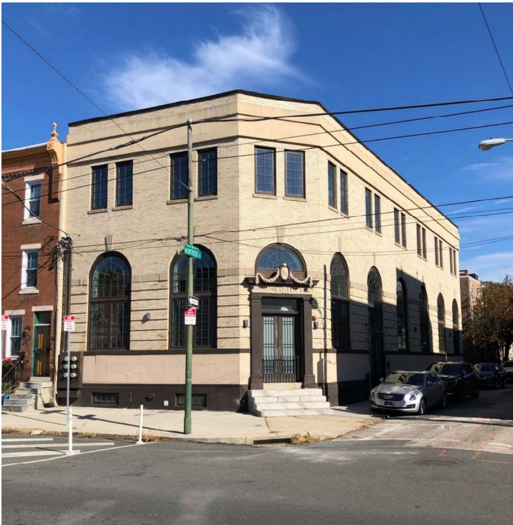
Figure 10: View of building from S. 11 th Street.
