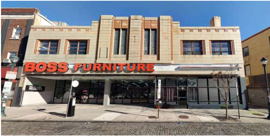
Figure 15: F.C. Woolworth building, 5607-13 Germantown Avenue, 1938. Source: Cyclomedia
