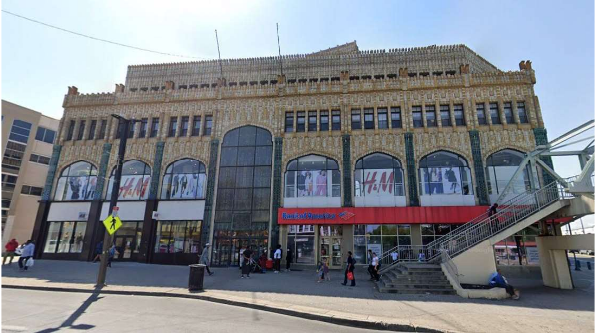
Figure 17: The McClatchy Building, George C. Nimmons, 2 S 69 th Street, Upper Darby, PA, 1926. Source: Google Streetview
