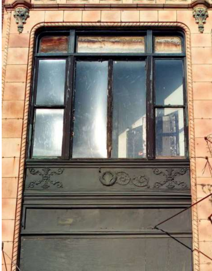
Figure 4. Window detail on 5131-37 Walnut Street, December 2022. Source: Cyclomedia
