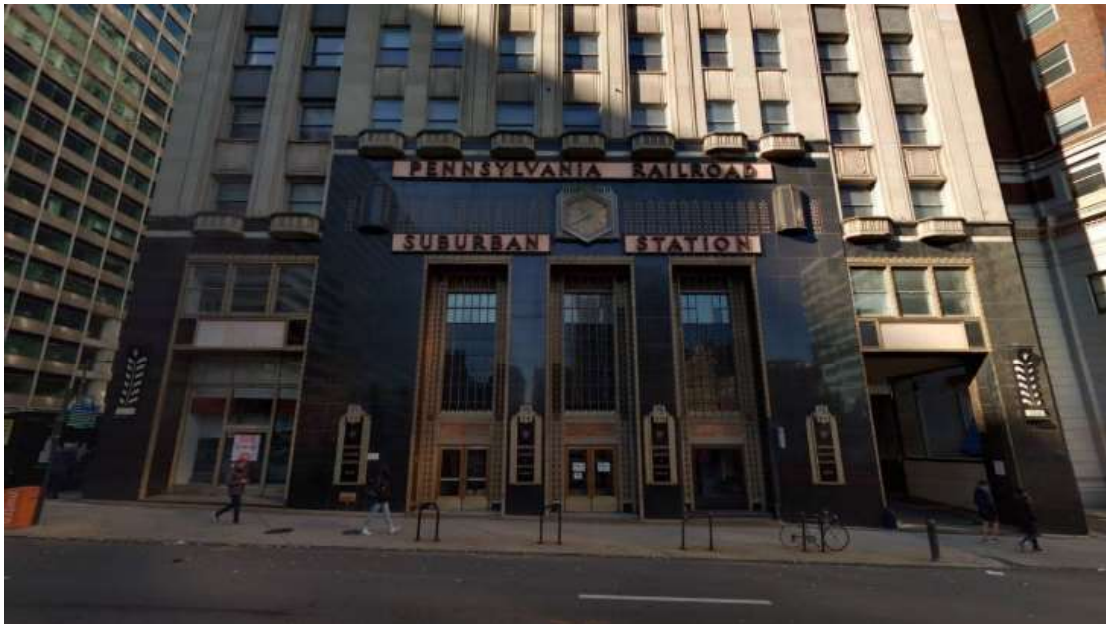
Figure 21: Suburban Station, 1601-29 John F. Kennedy Boulevard, 1930. Source: Cyclomedia
