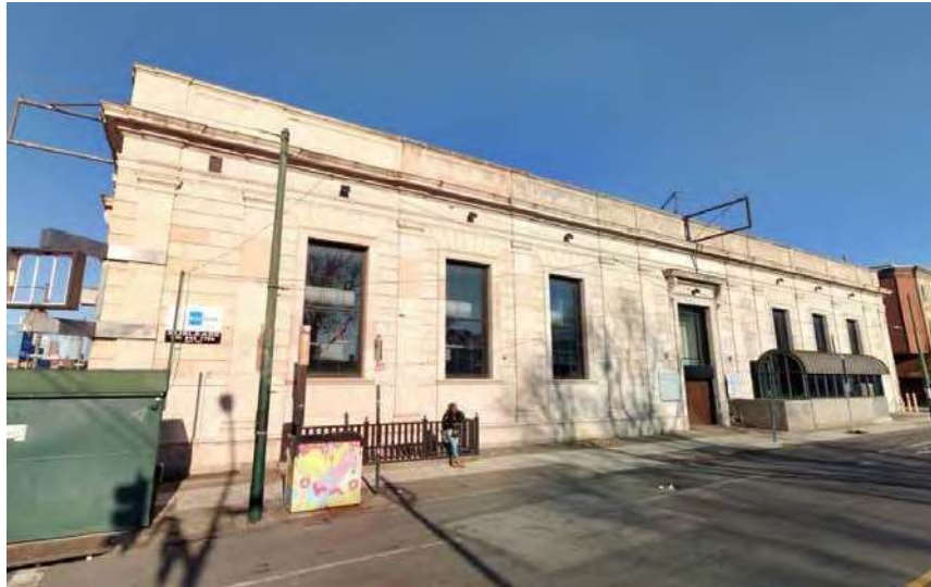
Figure 3: South elevation, looking northeast from Snyder Avenue.
