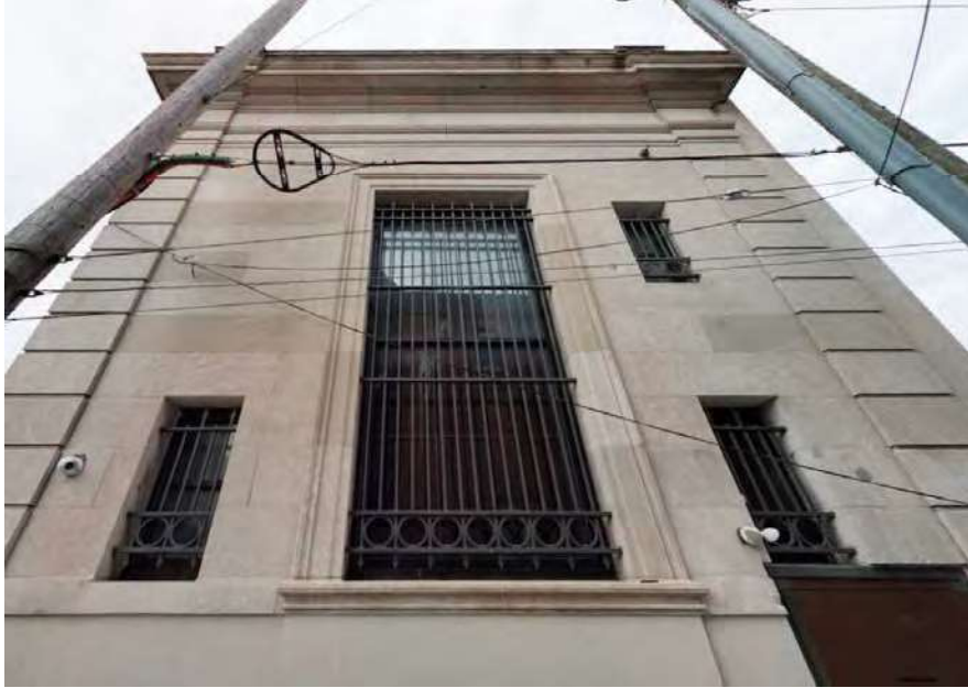
Figure 5: East elevation, looking west from Watts Street.
