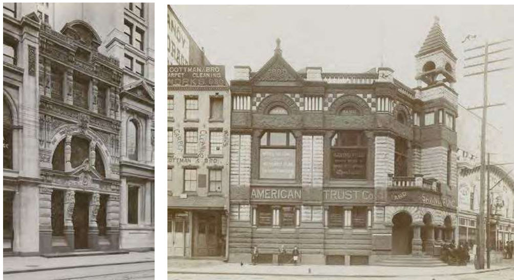
Figure 7 (left) - The Independence National Bank at 430 Chestnut Street, designed by Willis G. Hale and built in 1886 (Free Library of Philadelphia). Demolished.
