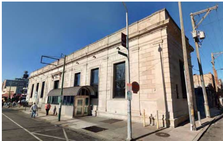
Figure 4: South elevation, looking northwest from Snyder Avenue.
