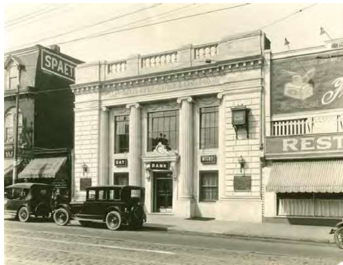
Figure 14 - The Lancaster Avenue Title & Trust Company at 3960 Lancaster Avenue, designed by Charles C. Schweiker and Charles H. Furster and built in 1923 (Indiana University Bloomington). Extant.
