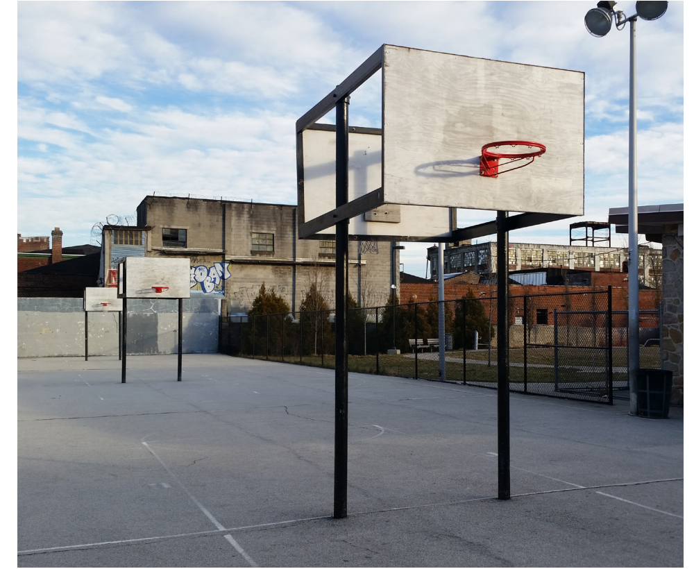
VIEW OF BASKETBALL COURTS ALONG LIPPINCOTT ST
