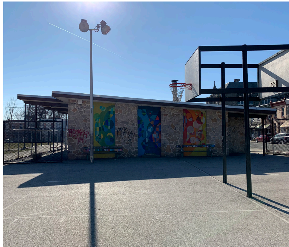
VIEW OF NORTH ELEVATION
