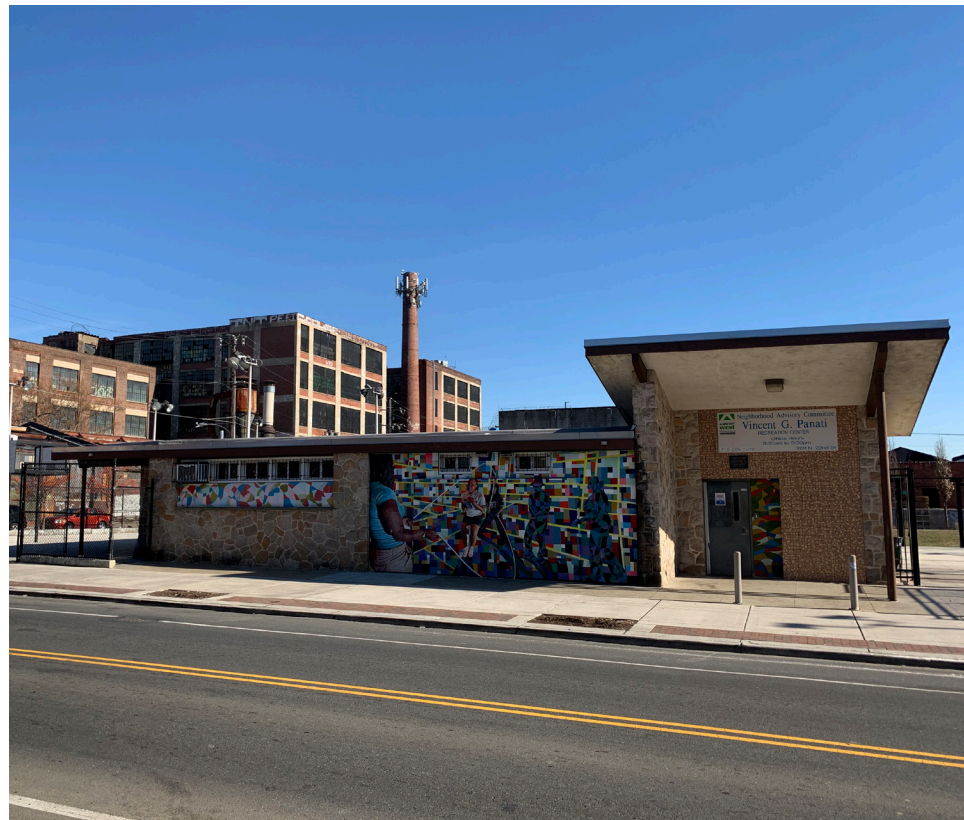
VIEW OF WEST ELEVATION
