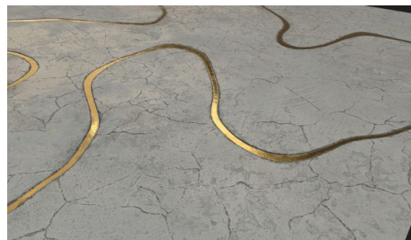
Brass Ground Detail Location: Motor Court & Sansom St
