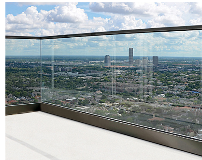
Glass Railing System Example Location: Typical Balcony Rails
