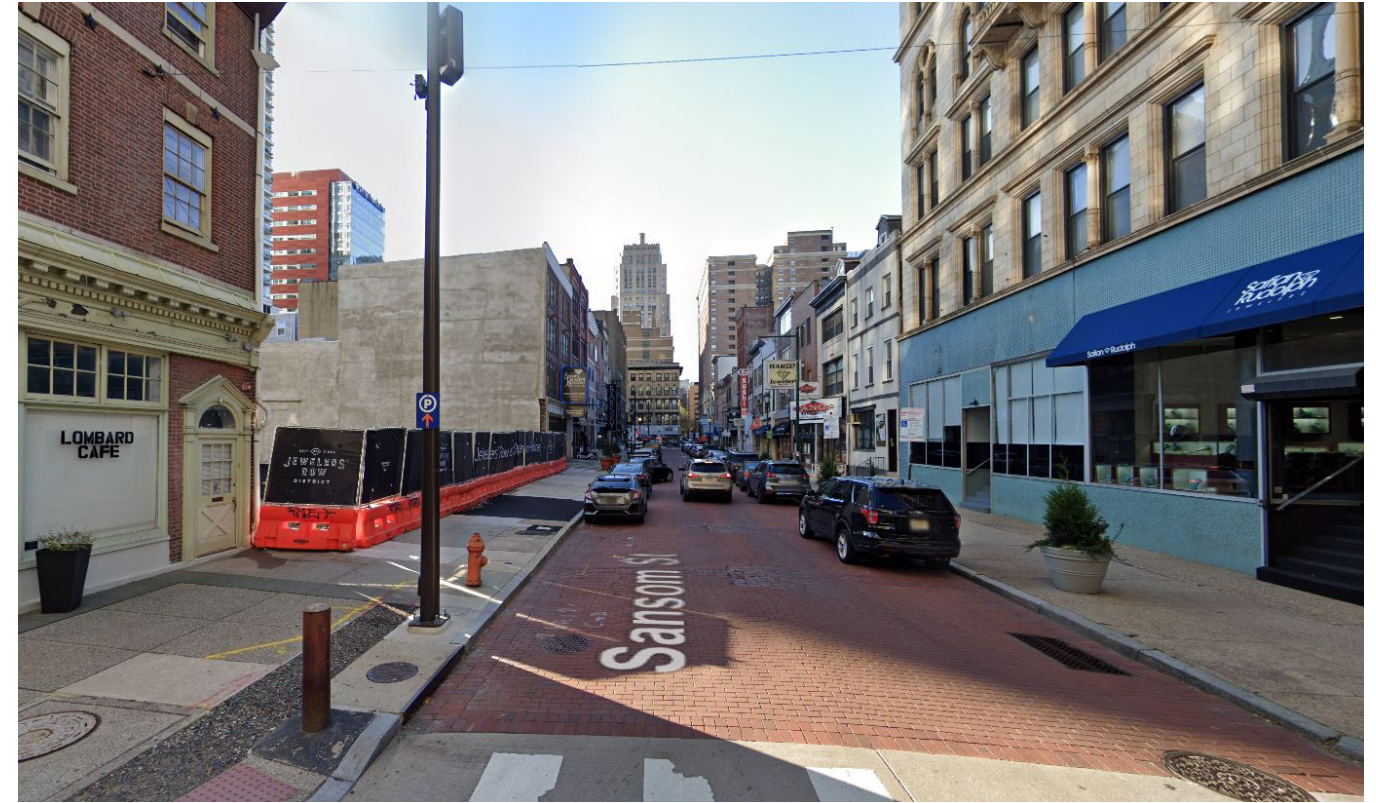
7 Looking West on Sansom St.
