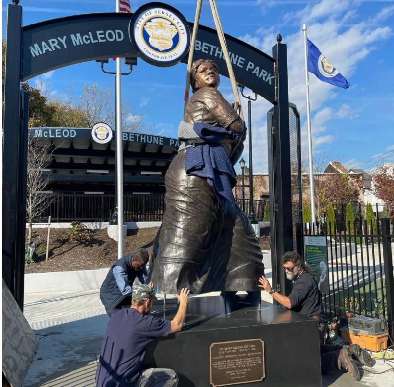
Example: Mary McLeod Bethune Monument Installation, NJ. 2021
