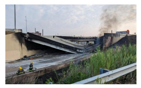
Highway collapse: The PFD responded to an intense fire caused by an overturned gasoline tanker-truck in June 2023. The intense flames and heat stemming from the fatal accident caused a portion of Interstate 95 to collapse in Northeast Philadelphia, closing the heavily traveled road for 12 days.
