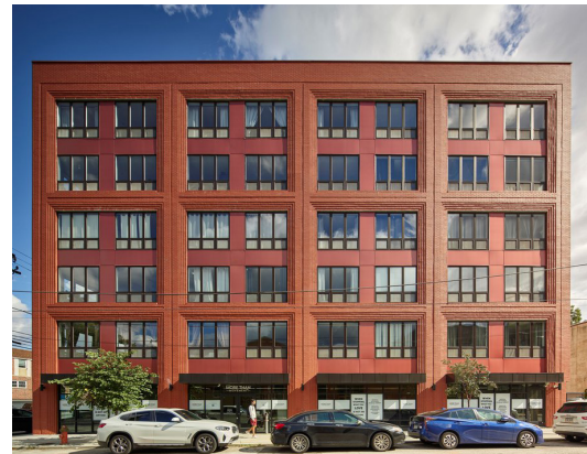
723 North 6th Street 35 Units, 39,400 SF Completed Spring 2021
