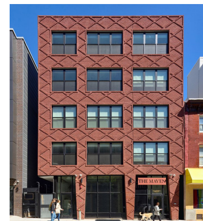
965 Frankford Avenue 33 Units, 38,700 SF Completed Spring 2021
