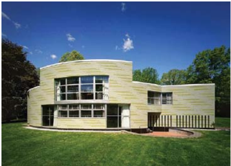
Brant House Robert Venturi Greenwich, CT 1972
