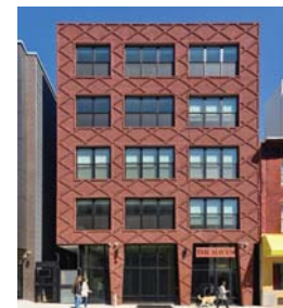
965 Frankford Avenue 33 Units, 38,700 SF Completed Spring 2021
