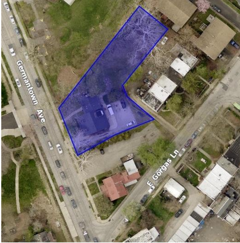
Figure 1a: 2022 aerial showing 6915 Germantown Avenue. Source: Atlas.
