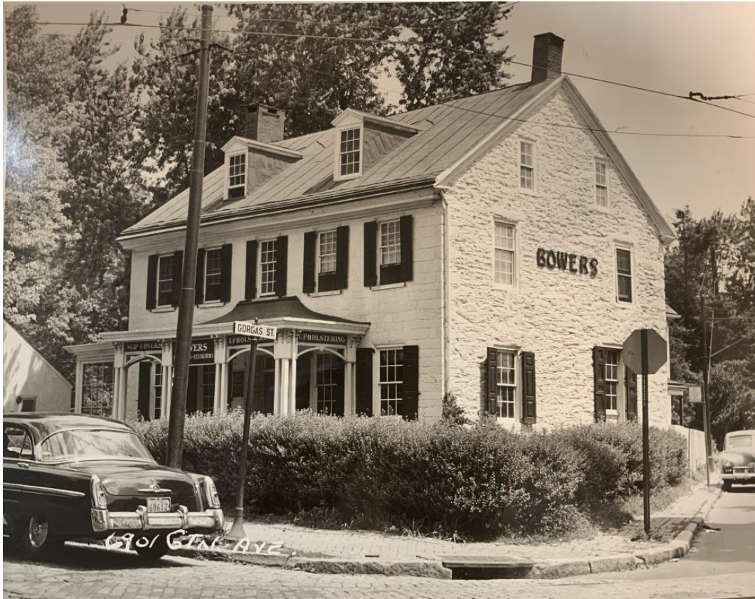
Figure 5: Historic photo of the property at the time of designation, June 1957. Source: Historical Commission files.
