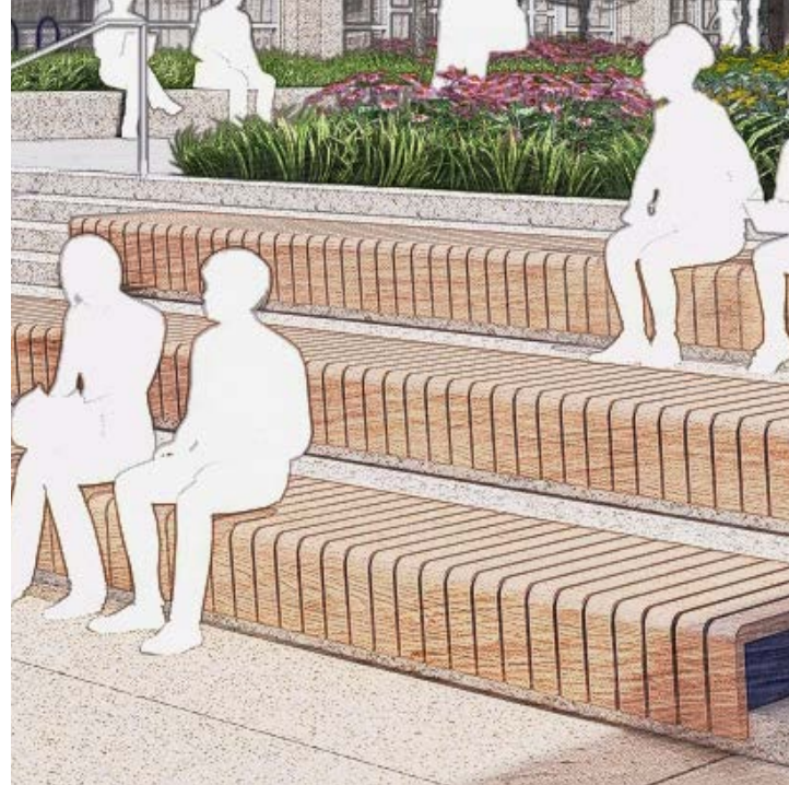
Wood seat tops on existing stairs
