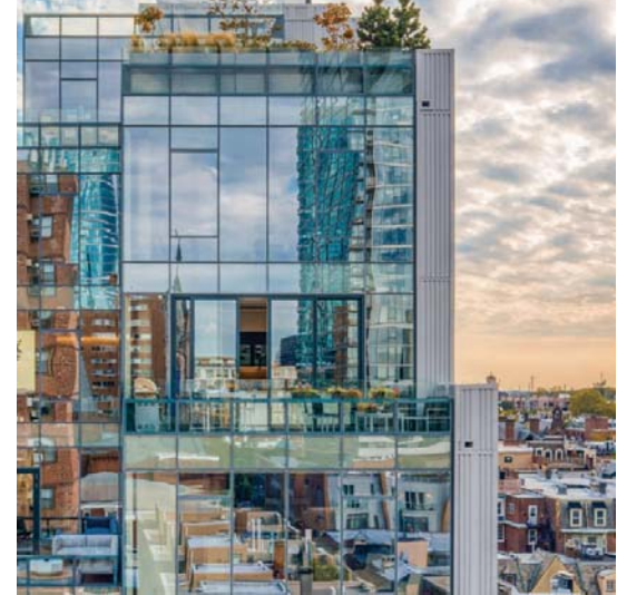
3 4 Window Wall System with Spandrel
