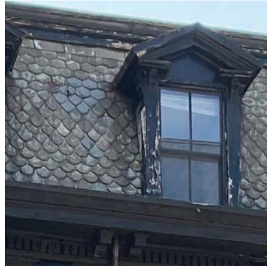
6 Existing Slate Shingles to be Restored
