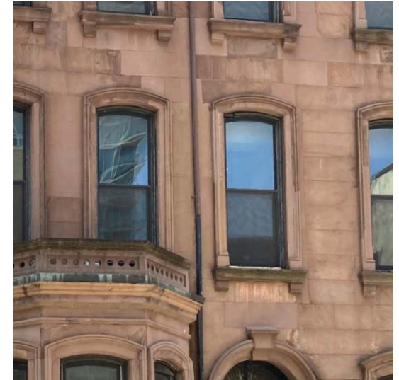
8 Existing Masonry to be Restored
