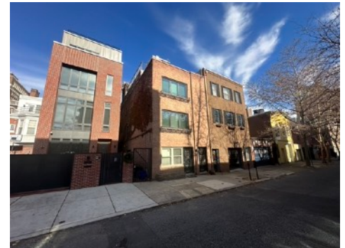
New Construction North Side
