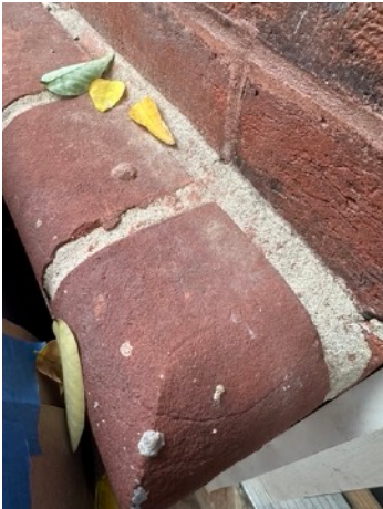
View of 1950's brick should marble be removed — Size & color of brick is different & width of joints is double compared to historic brick above.
