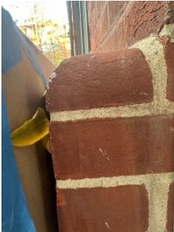
Exploration of brick and basement window opening (RIGHT) revealed that brick is interconnected with a rubble foundation and supporting steel that was installed when the house was converted to a duplex. Contractors deemed it unsafe to remove.
