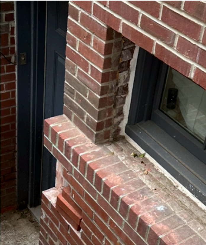
Exploration of brick and basement window opening (RIGHT) revealed that brick is interconnected with a rubble foundation and supporting steel that was installed when the house was converted to a duplex. Contractors deemed it unsafe to remove.
