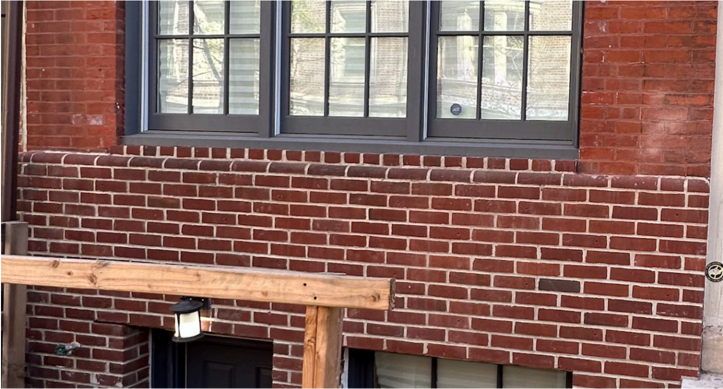
View of 1950's brick should marble be removed — Size & color of brick is different & width of joints is double compared to historic brick above.
