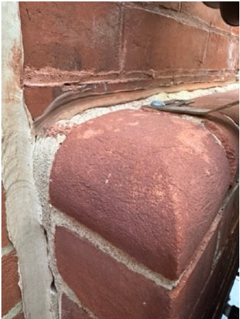
Exploration of brick and basement window opening (RIGHT) revealed that brick is interconnected with a rubble foundation and supporting steel that was installed when the house was converted to a duplex. Contractors deemed it unsafe to remove.
