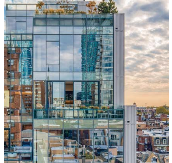
3 4 Window Wall System with Spandrel
