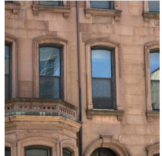
8 Existing Masonry to be Restored
