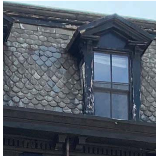
6 Existing Slate Shingles to be Restored
