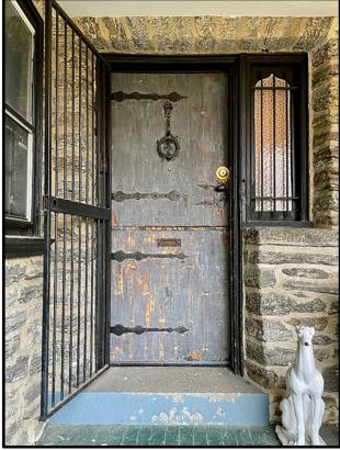
Figure 8. The entry Dutch door and Tudor-arched side light in the recessed entry porch.
