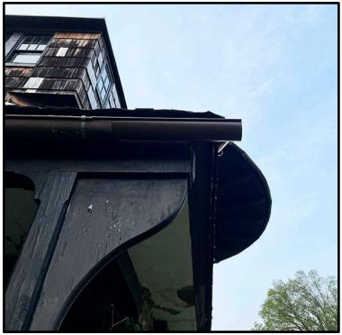
Figure 7. The curvaceous brackets at the rear porch assembly.
