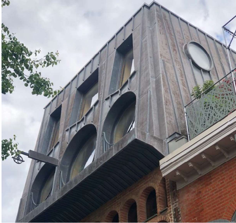
Figure 9: The front of the mansard features oversized rounded arch and pentagonal window openings. A pulley system is installed and projects outward. While the pulley may have been a practical tool for moving large items to the upper levels, it is also a nod to the past.
