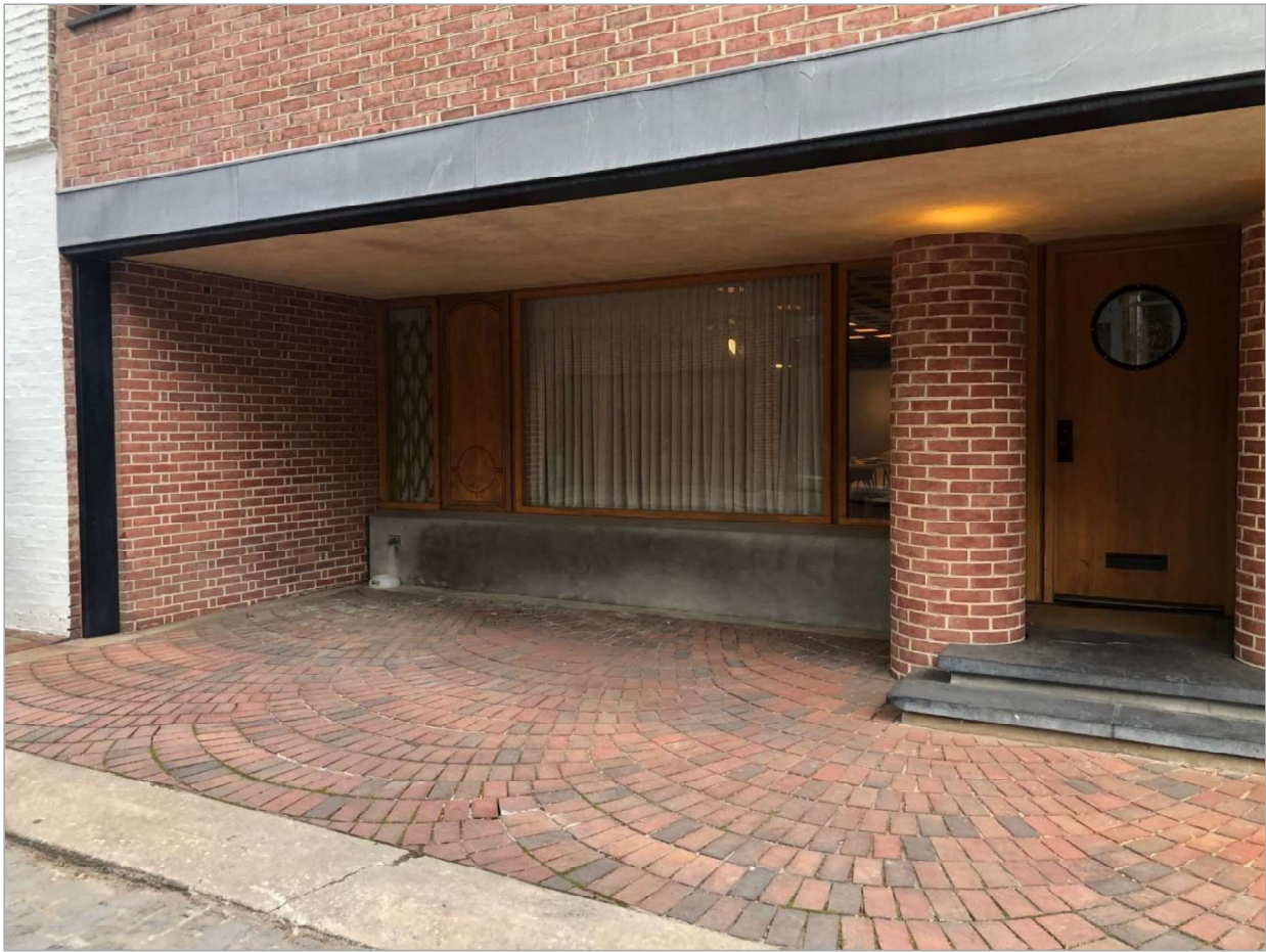
Photograph of exterior first level. Property owner Andrea Hemmann confirmed the semi-circular paving pattern was designed by Frank Weise.
