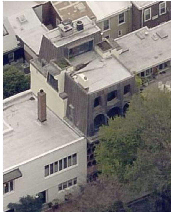
Figure 14: A view showing the top of the front facade and roof mezzanine. The top of the mansard has a flat roof.
