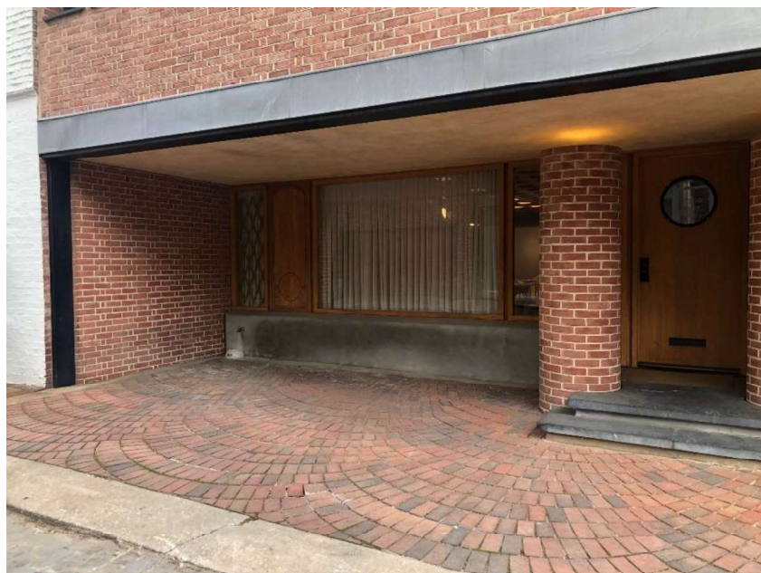
Figure 8: The recessed open space on the first floor was designed as a carport and main entrance area. The inset wall contains a picture window and two entry doors. The semi-circle paving pattern was designed by the architect.
