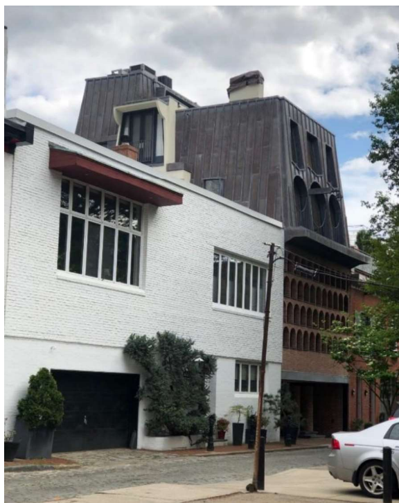
Figure 2: View looking south down S. Chadwick Street. The mansard rises prominently above the neighboring buildings. The chimney, Juliet balcony, and roof mezzanine on the building's north wall are visible from street level.
