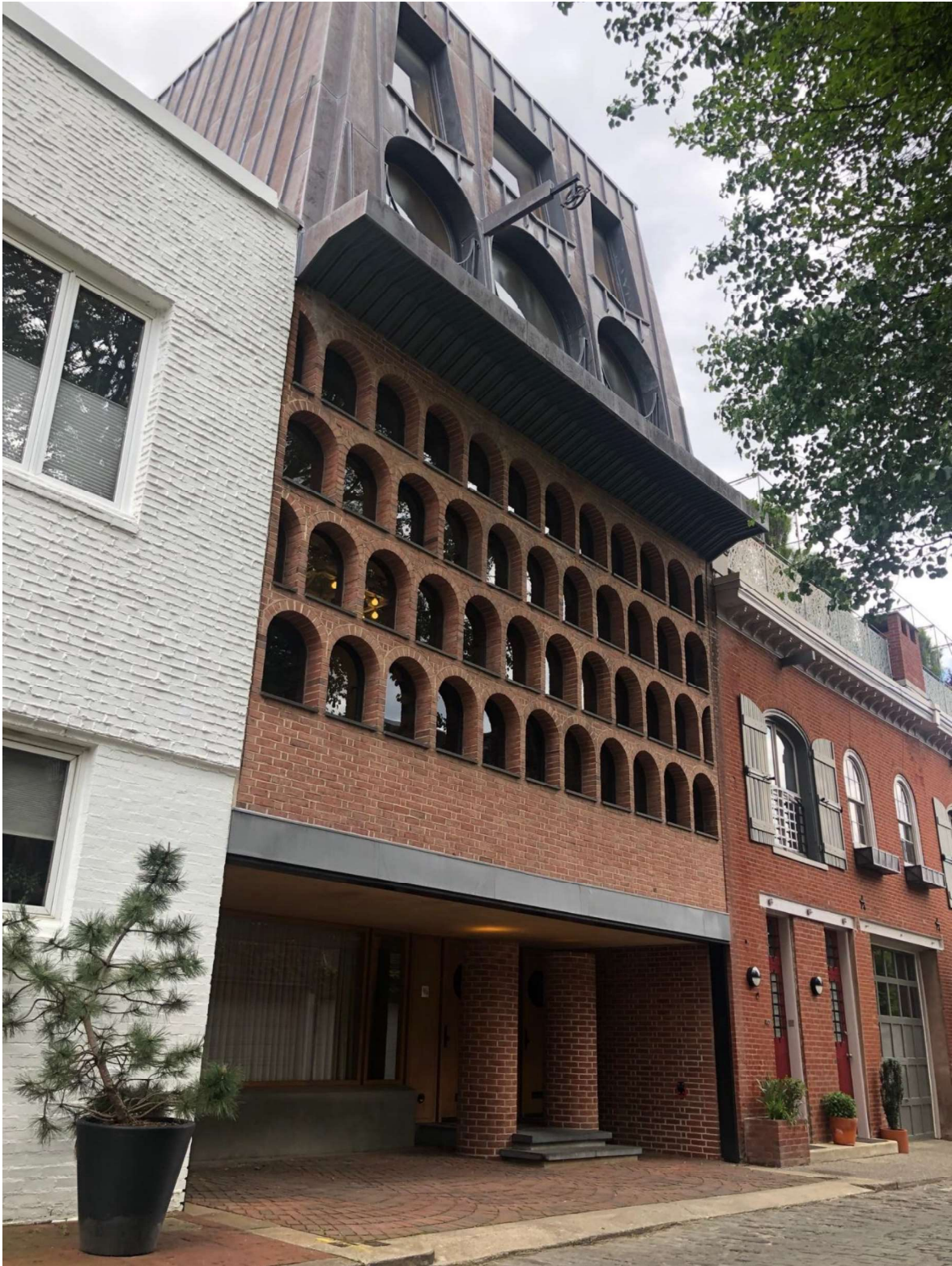
Figure 4: A full view of the front façade. Weise's skill with Modernist residential design is seen on the first floor. He sets the wall and entrance back to create a shadowed area at the building's base. This encourages a visual illusion of the upper levels floating above.
