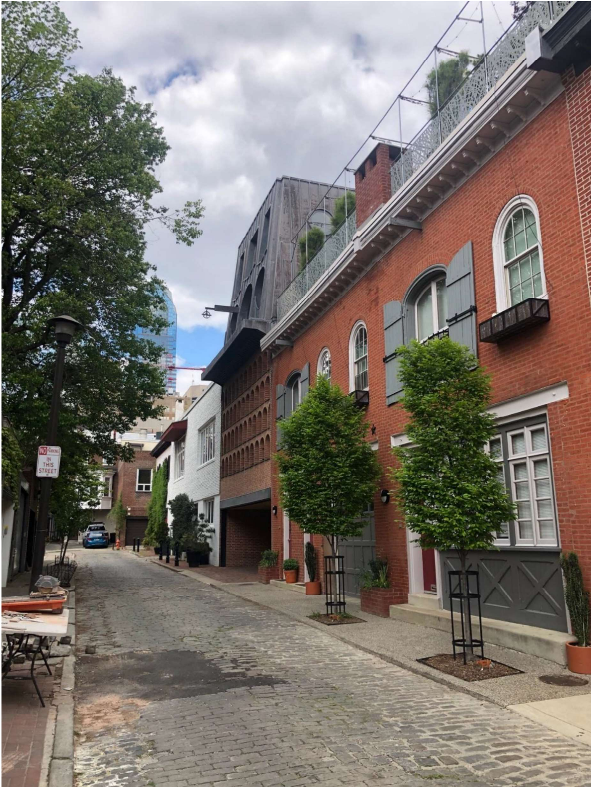
Figure 5: View looking north up S. Chadwick Street toward the intersection with Cypress Street. The east side of the street was developed in the nineteenth century primarily with two-story stables. The original stable at 307 S. Chadwick Street was never fully demolished. Party walls and floors (and joists) appear to have been incorporated into the altered building.
