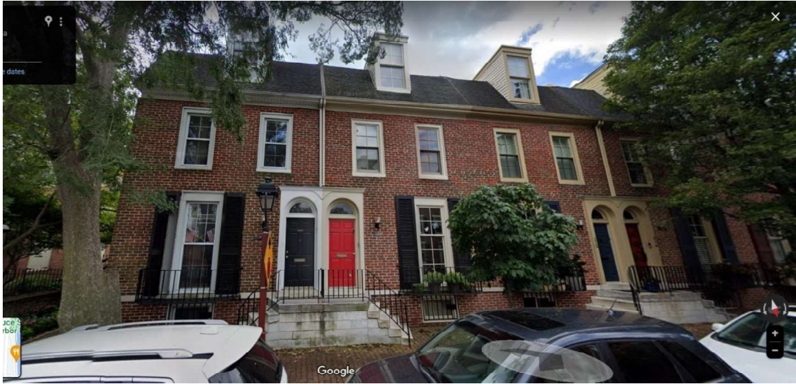
Figure 44: Rowhouse block, 1965. 208-26 Pine St, Philadelphia PA. Photo credit: Google Street View.
