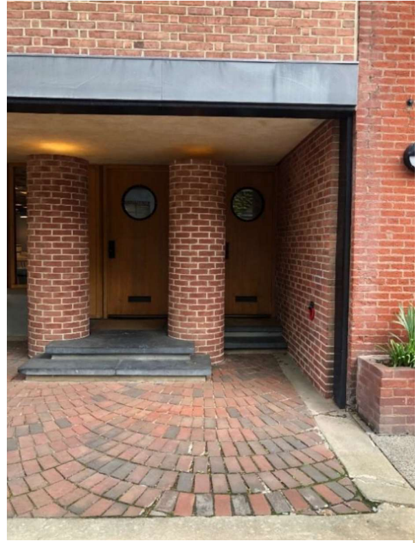
Figure 7: The two entrances are accessed by blue stone steps. The entry doors are wood with circular windows. Separate entryways for the studio and living areas allowed for privacy between the spaces.
