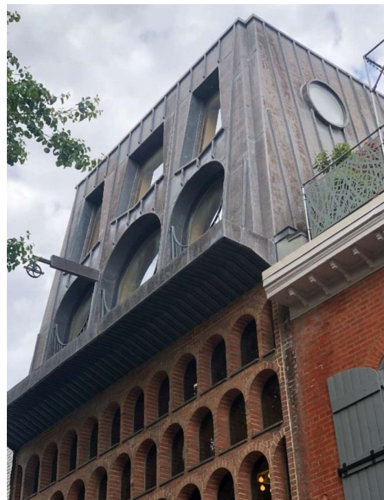
Figure 3: The mansard's front façade features oversized window openings made up of a one row of arches and an upper row of pentagons. A port hole window on the south façade was a later alteration by the architect.
