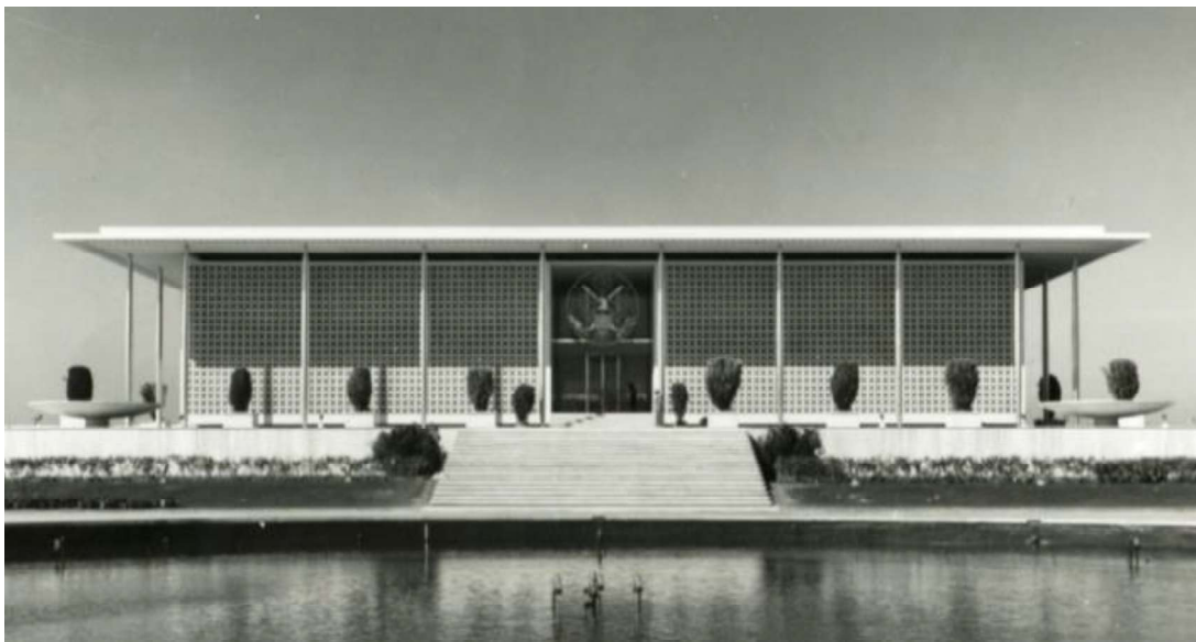
Figure 45: U.S. Embassy New Delhi, India. Completed 1959. Architect Edward Durrell Stone. Photo credit: Docomomo US, https://www.docomomo-us.org/register/u-s-embassy-in-new-delhi .
