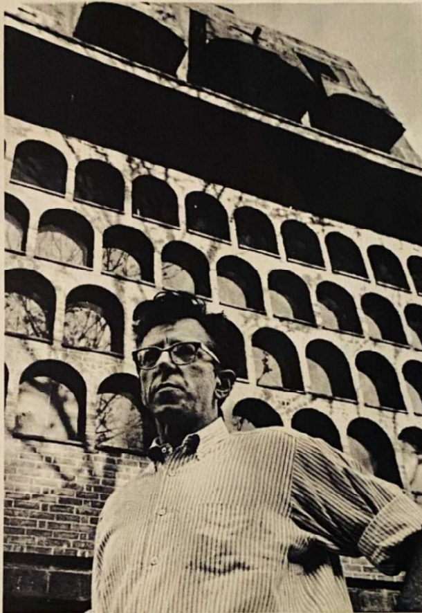
Frank Weise stands proudly in front of his imposing unfinished architectural dream.
