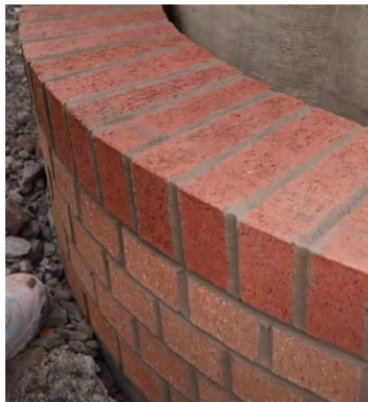
2 RAISED BRICK PLANTER: 2'H RED BRICK CURVED PLANTER CONTAINING SMALL ORNAMENTAL TREES
