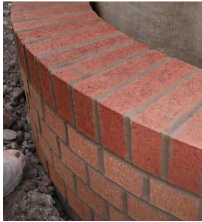
3 CURVED BRICK CORNERS OF RAISED PLANTER WITH ROWLOCK COURSE
