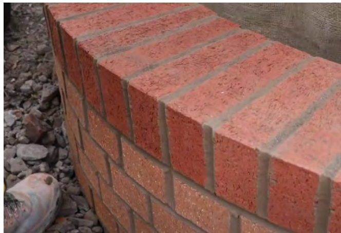
RAISED PLANTER WALL USING BRICK TO MATCH ARCHITECTURE WITH TOP ROWLOCK COURSE
