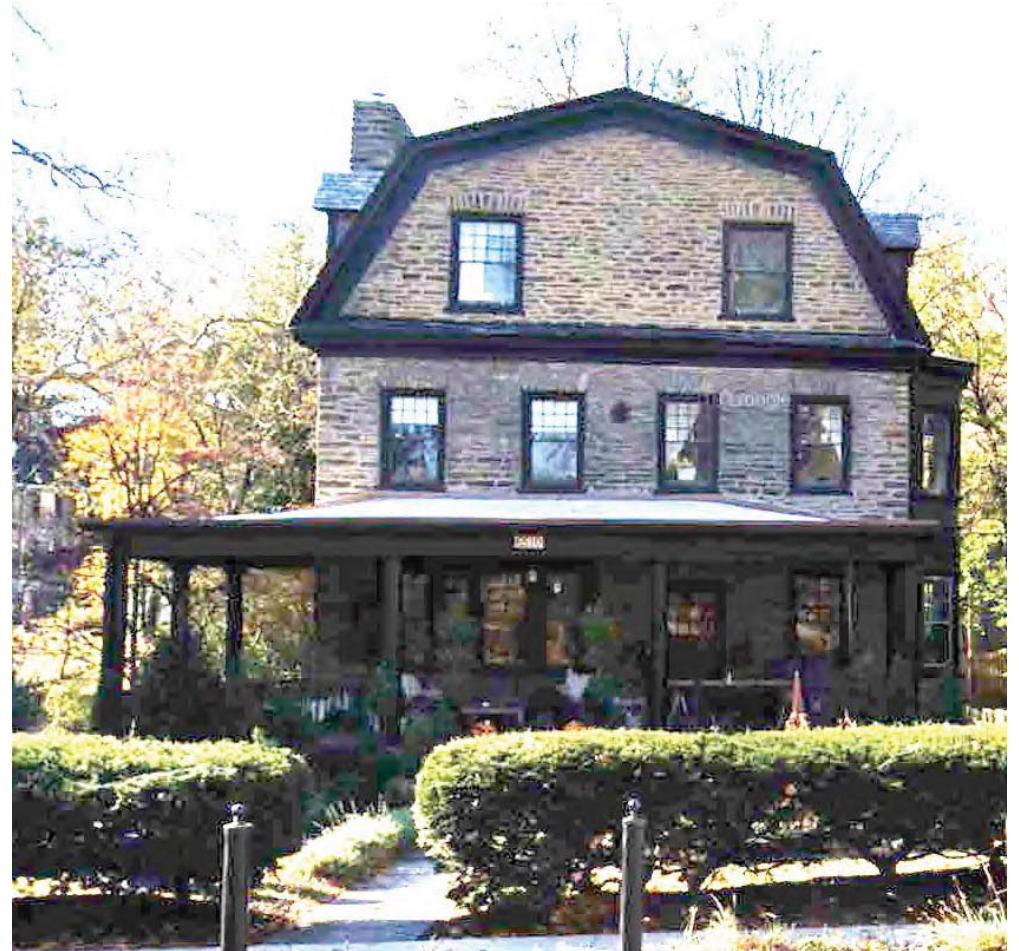
6500 block Lincoln Drive coursed quarry-faced rubble Jack arches over windows
