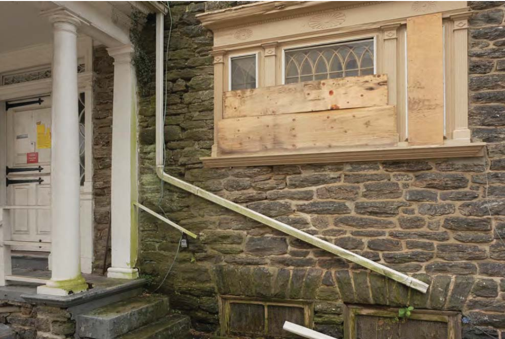
Off-the shelf details: Porch columns, triple window
