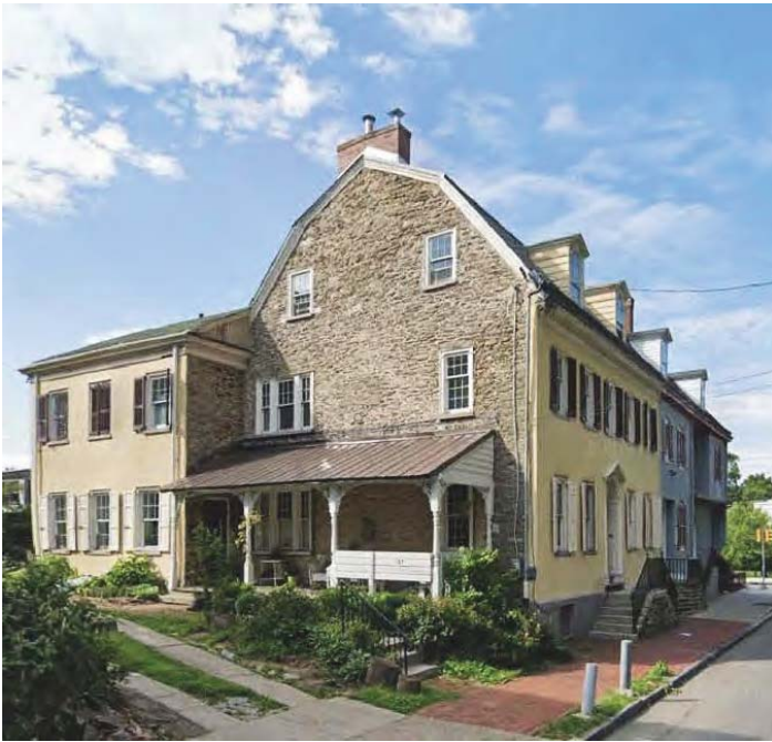
125 W. School House Lane Historic straight gambrel roof
