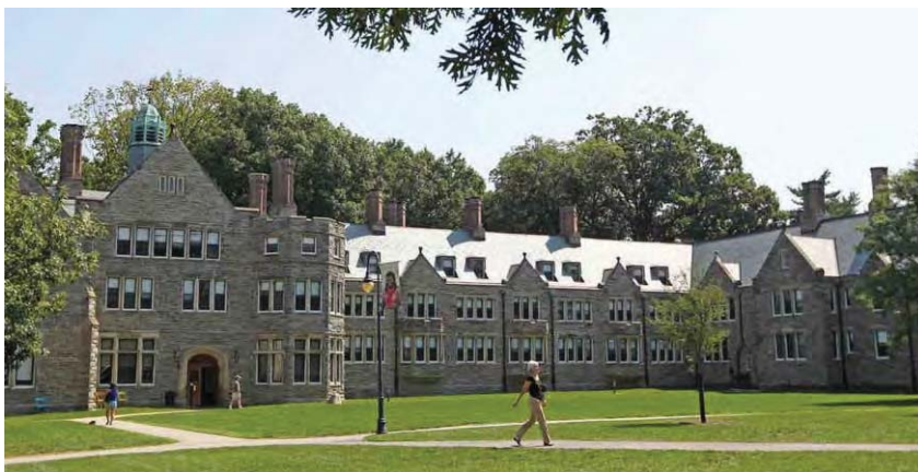
Cope and Stewardson, Denbigh Hall (1890-1) with full Gothic Revival style, limestone, clustered chimneys, buttressed corners
