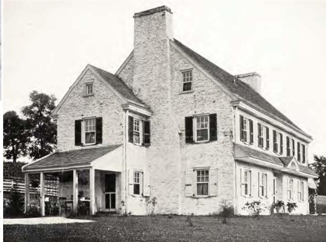
Duhring, Okie & Ziegler, Philander Knox House, c. 1905 Stonework, details, pent eave, cornice does not continue on gable end, rough cast barn stucco on rubble stone, simple square post porch
