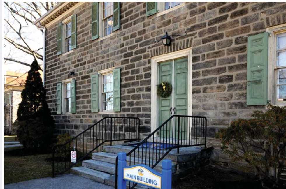
Main Building Among earliest buildings recorded by Historic American Buildings Survey
