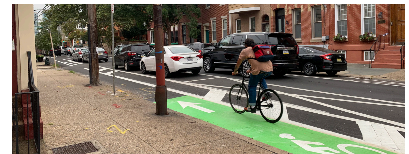
Parking separated bikeway on a one-lane one-way street, 22nd Street
