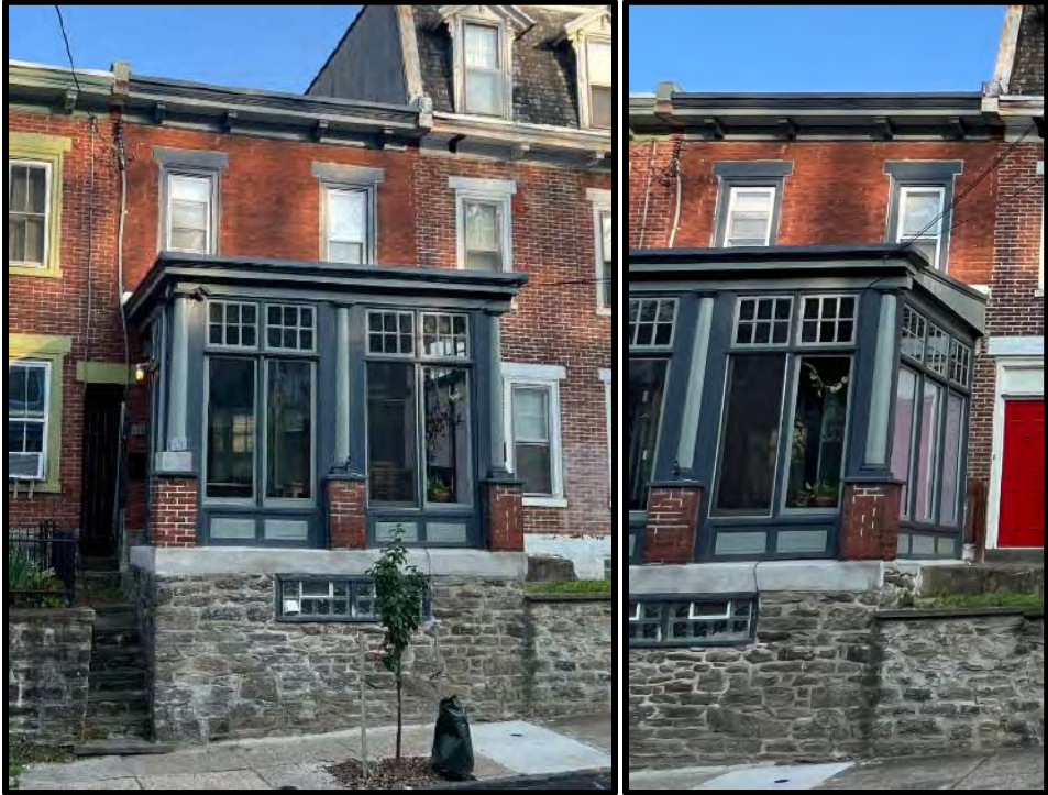
The NW and SW elevations. Source: Keeping Society of Philadelphia, 2023.
