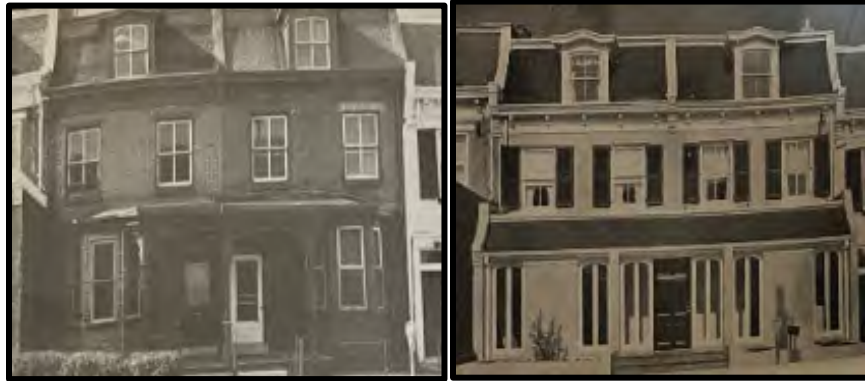
Figure 70. “Before and After” photographs of 39 East School House Lane, which was converted from two private houses to the office of Hassinger and Schwam, Architects. Source: Jack Hornung. “Rebuilding Germantown, A Progress Report...,” Unknown Publication, March 1965. From the records of GHS.
