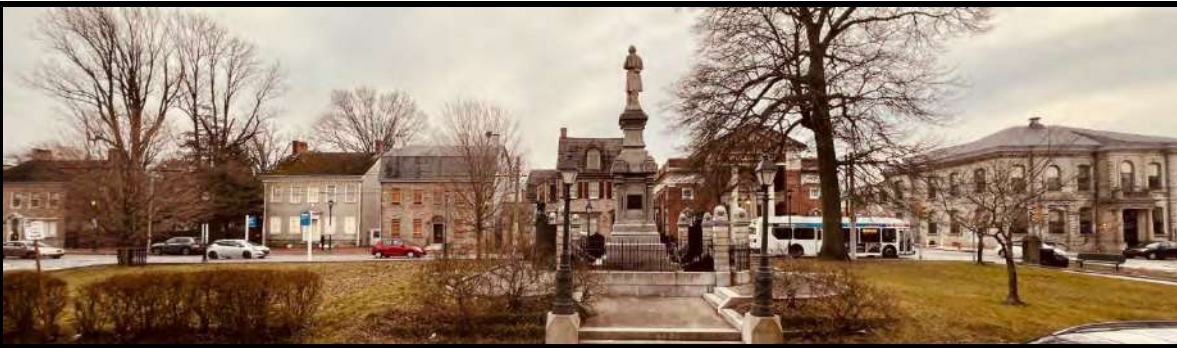
Figure 5. Top: Looking north, the Fromberger Houses at 5503 and 5505 Germantown Avenue and the Market Square Presbyterian Church at 5507-17 Germantown Avenue. Figure 6. Middle: Looking southwest, the Deshler-[Franks]-Morris House at 5442 Germantown Avenue; the Bringham House at 5448 Germantown Avenue; and the Thomas Armatt House at 5450 Germantown Avenue. Figure 7. Bottom: Looking southwest, the "west" side of Market Square from across the actual Market Square with the Soldiers' Monument at the center. Source: Oscar Beisert, 2023.
