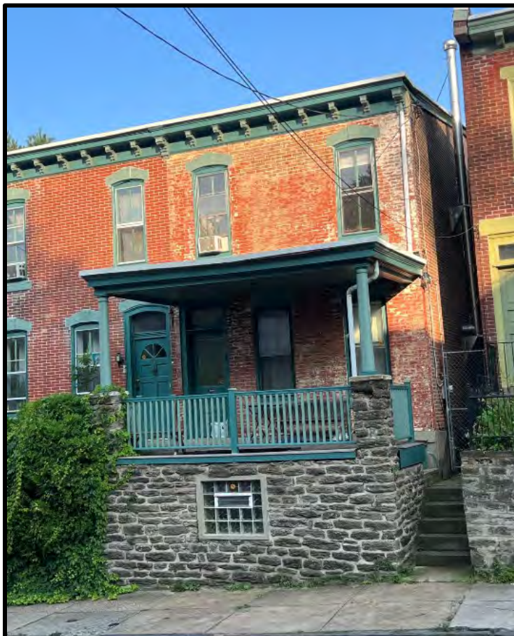
The NW and SW elevations. Source: Keeping Society of Philadelphia, 2023.
