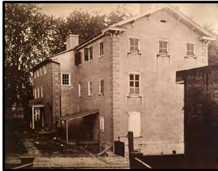
Figure 54. “This is the first steam grist mill erected in the township of Germantown, owned by Wyndham H. Stokes.” Built in 1838, Stokes’ Mill (Demolished) at 45 Church Lane opposite the subject property eventually became the hall of Seminole Tribe, No. 30, Improved Order of Red Men, and was later demolished for a new building. Source: “Historical Relics.” Public Ledger , Undated, Shoemaker Collection, HSP.
