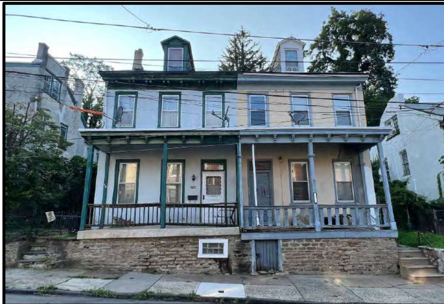
Top: The SE and NE elevations. Bottom: The SE elevation. Source: Keeping Society of Philadelphia, 2023.
