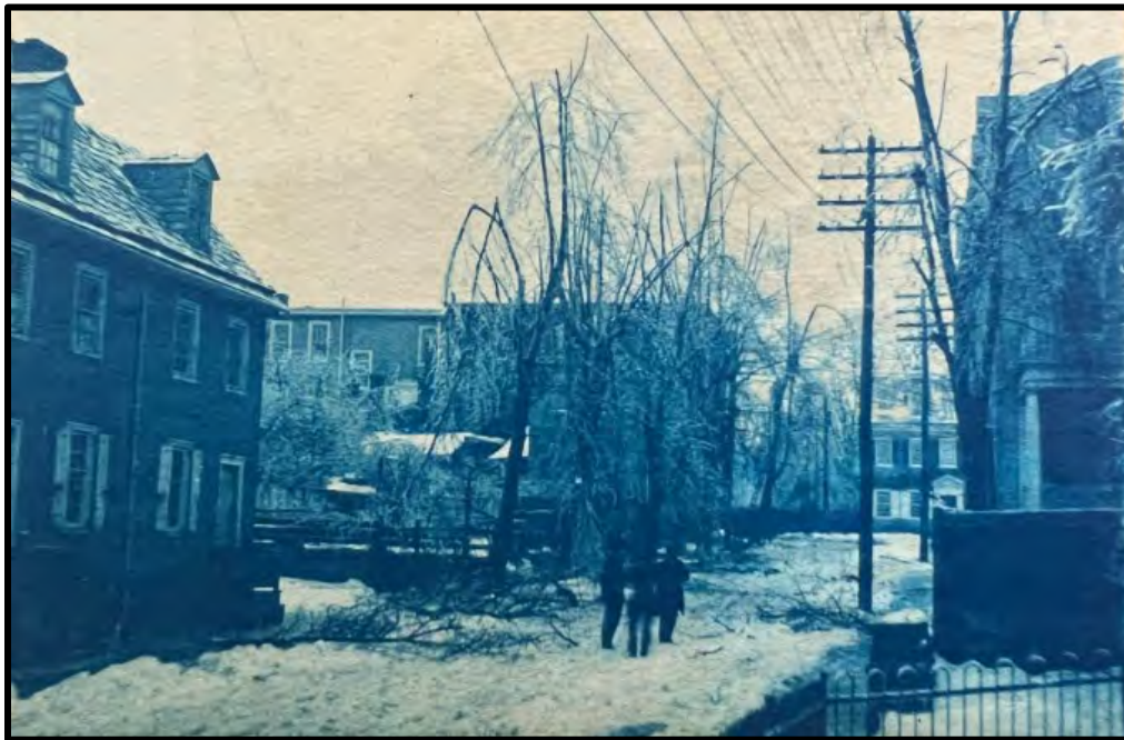
Figure 78. Looking up Church Lane towards Market Square with the Deshler-[Franks]-Morris House visible in the background. Source: GHS.
