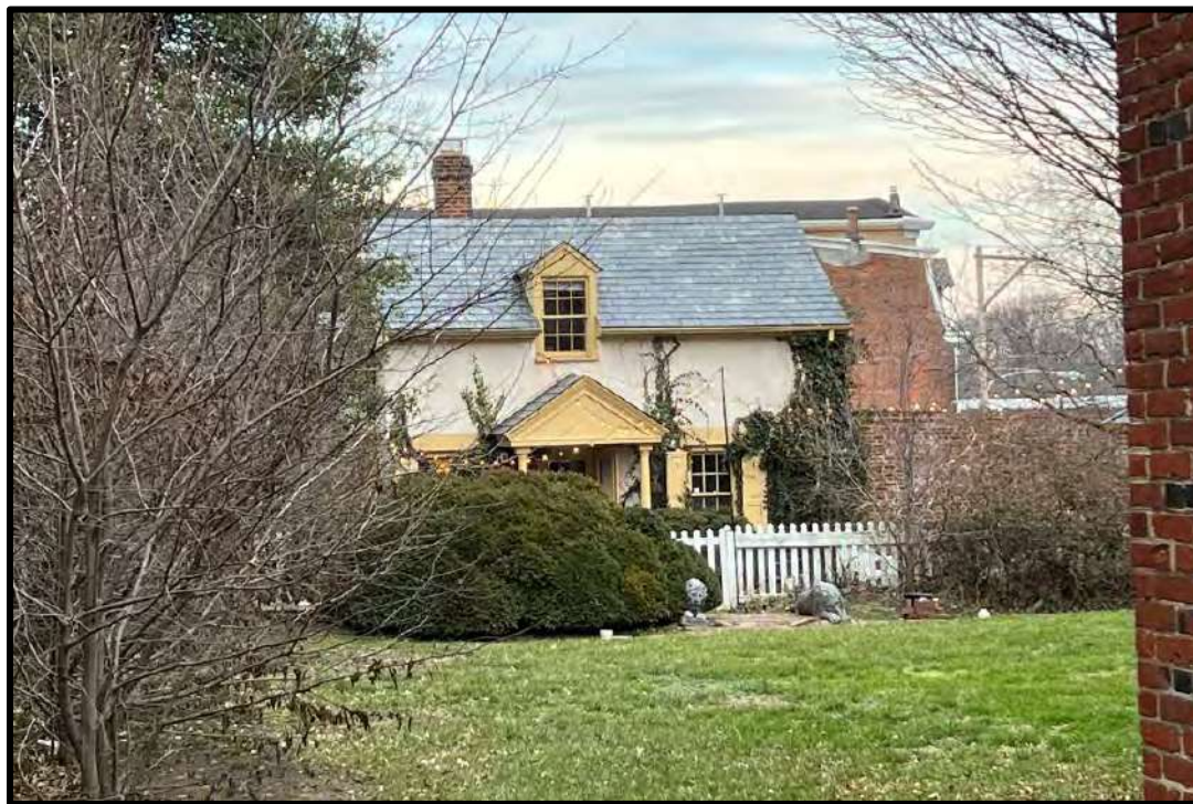
Cottage/Janitor's Lodge, 5503-05 Germantown Ave., SW Elevation. Source: Oscar Beisert, 2022.
