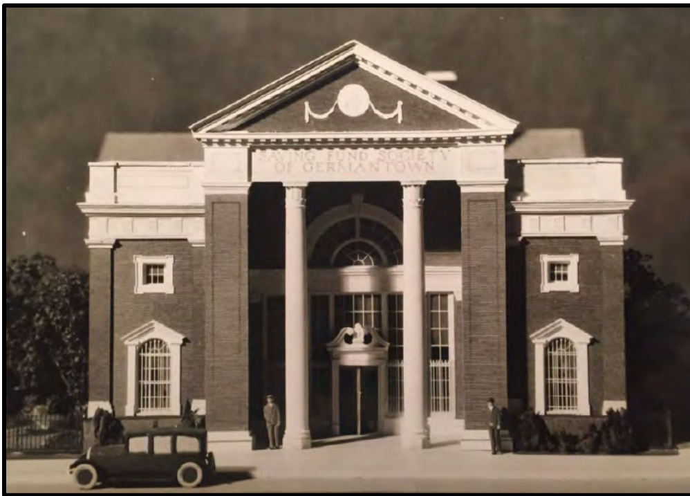
Figure 42. A model of the Saving Fund Society of Germantown's new building in 1929. Source: GHS.
