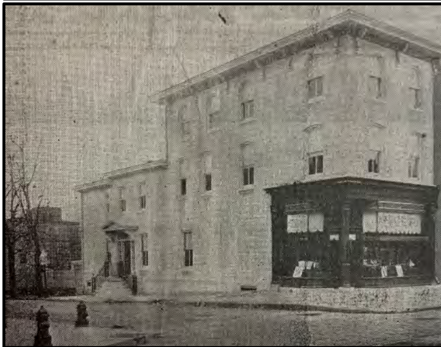
Top: The Charles L. Eberle Pharmacy, 5443-45 Germantown Ave., NW and SW Elevations. Source: Oscar Beisert, 2023. Bottom: The Charles L. Eberle Pharmacy, 5443-45 Germantown Ave., NW and SW Elevations, ca.1910. Source: GHS.
