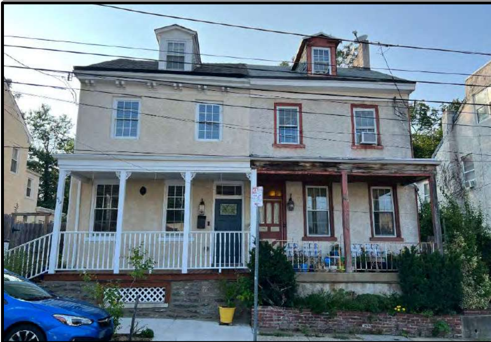
Top: The SE and NE elevations. Bottom: The SE elevation. Source: Keeping Society of Philadelphia, 2023.
