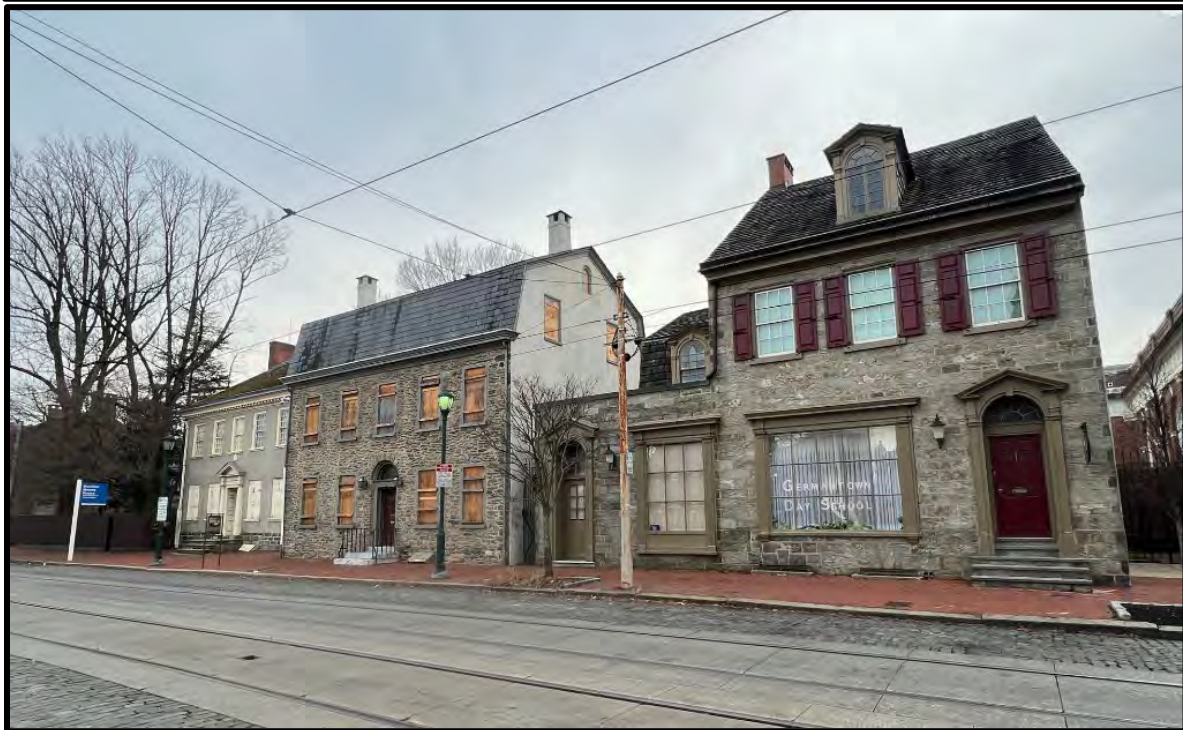
Top: Deshler-[Franks]-Morris, Bringhurst, & Armat Houses, NE Elevation. Bottom: The Deshler-Morris, The Bringhurst, & the Armat House, NE and NW Elevations. Source: Oscar Beisert, 2023.
