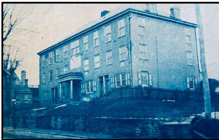
Figure 64. Philomathean Hall, East Wister Street, showing the central entrance to the third-floor lodge rooms, and the doors flanking the central entrance that led to the four row houses that subsidized the cost of the building. Source: GHS.
