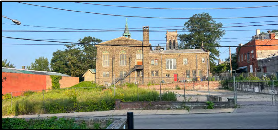
Looking SE, Vacant Lot, 26-34 Church Lane. Source: Keeping Society of Philadelphia, 2023.
