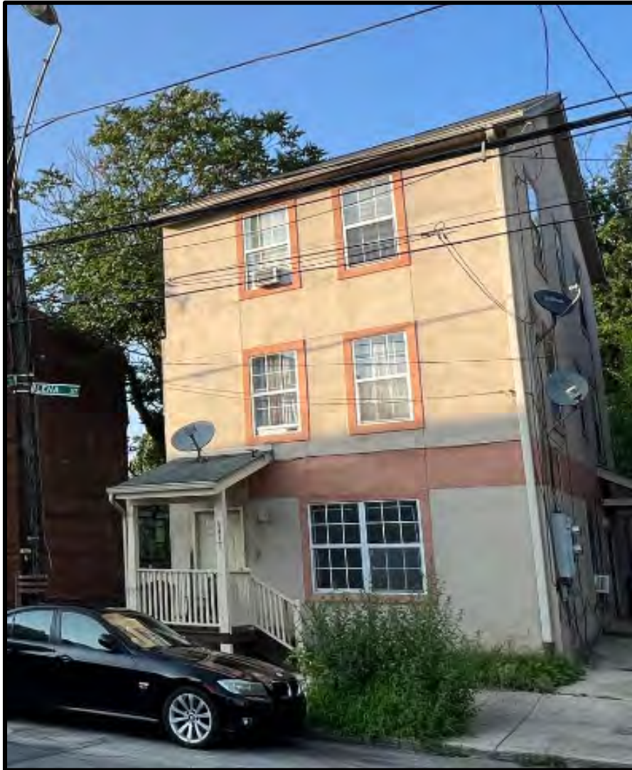
The SW and SE elevations of the subject property. Source: Keeping Society of Philadelphia, 2023.
