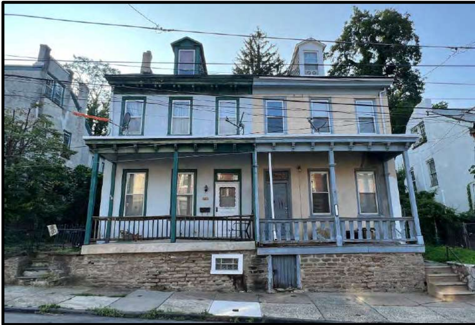
Top: The SE and SW elevations. Bottom: The SE elevation. Source: Keeping Society of Philadelphia, 2023.
