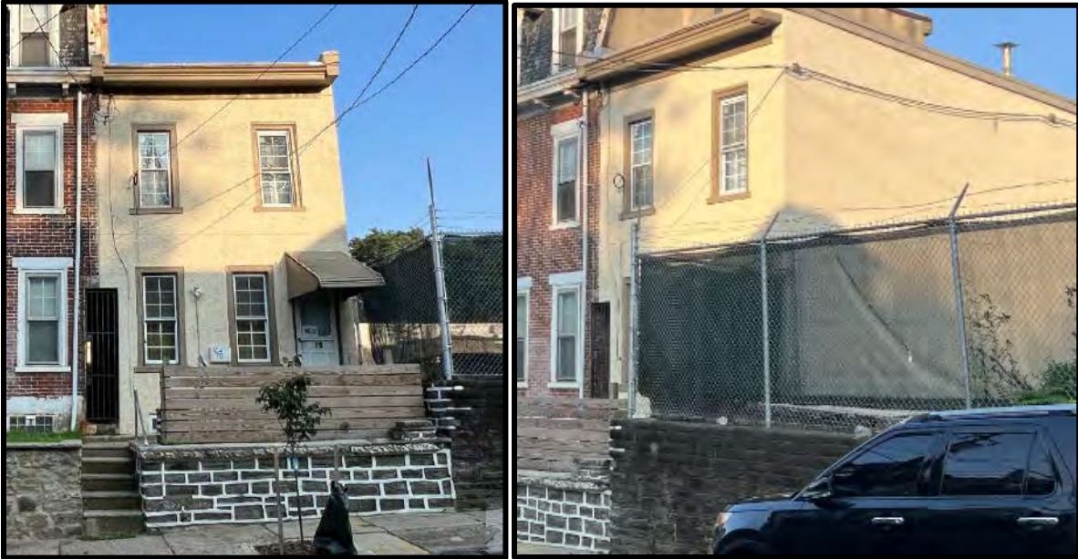
The NW and SW elevations. Source: Keeping Society of Philadelphia, 2023.
