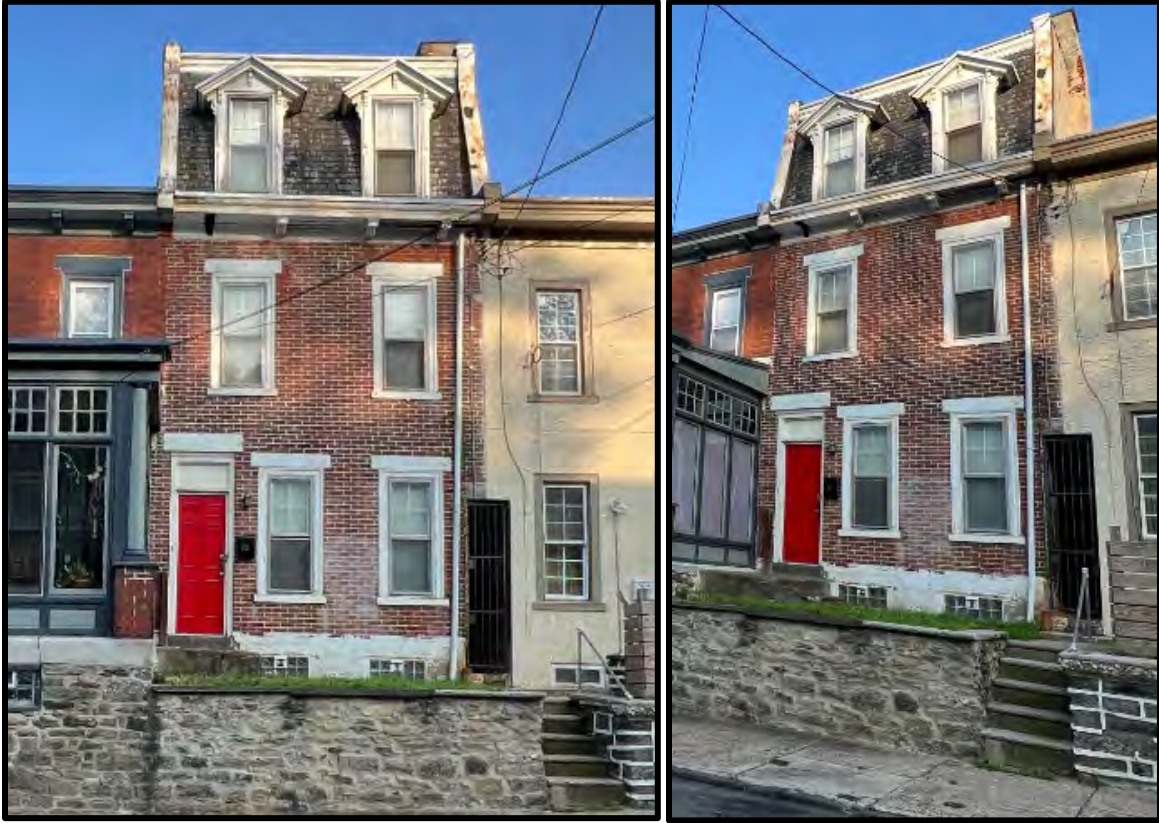
The NW and SW elevations. Source: Keeping Society of Philadelphia, 2023.
