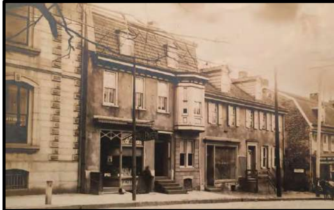
Top: Commercial Building, 5506 Germantown Ave., NE Elevation. Source: Oscar Beisert, 2023. Middle left: Commercial Building, 5506 Germantown Ave., NE Elevation, after 1909. Middle right: Rendering of Commercial Building, 5506 Germantown Ave., NE Elevation, ca.1909. Source: GHS. Bottom: Earlier Store-and-Dwelling (Demolished), 5506 Germantown Ave., NE Elevation, before 1909. Source: Shoemaker Collection, HSP.
