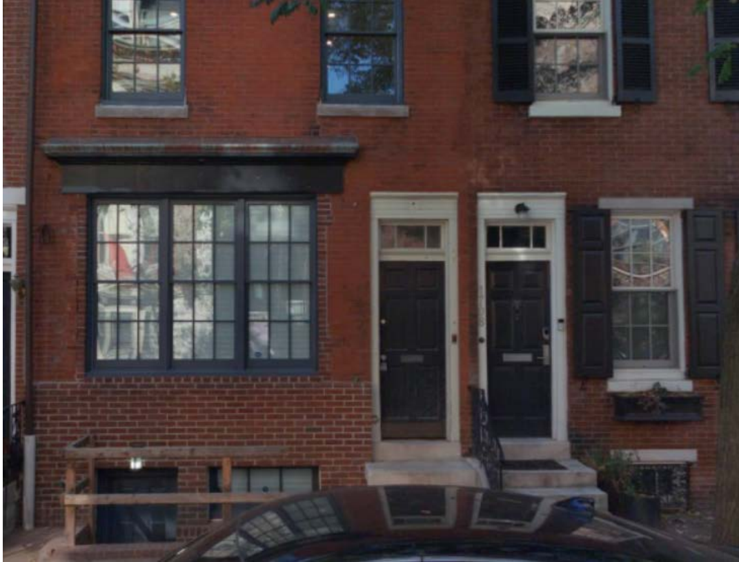
Figure 2. November 2022, with approved windows installed but no water table or doorway alterations.
