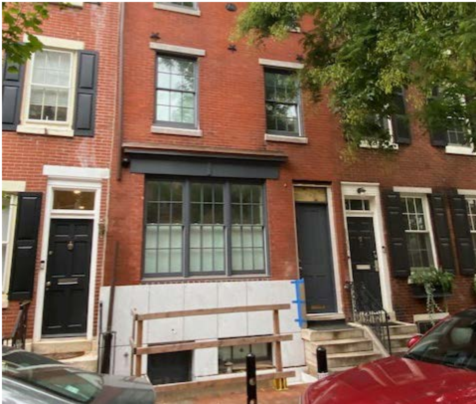
Figure 3. September 2023, work in progress.
