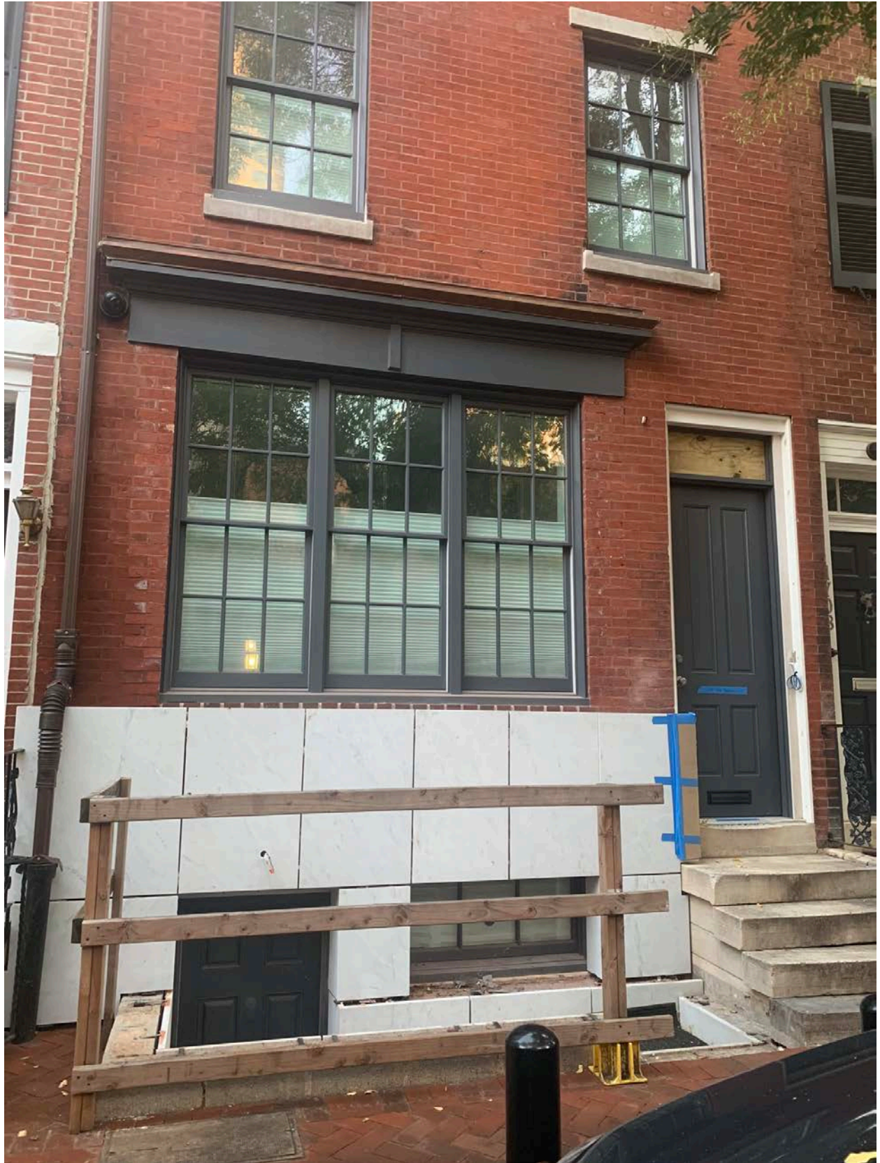
Figure 6. October 2023, work in progress.
