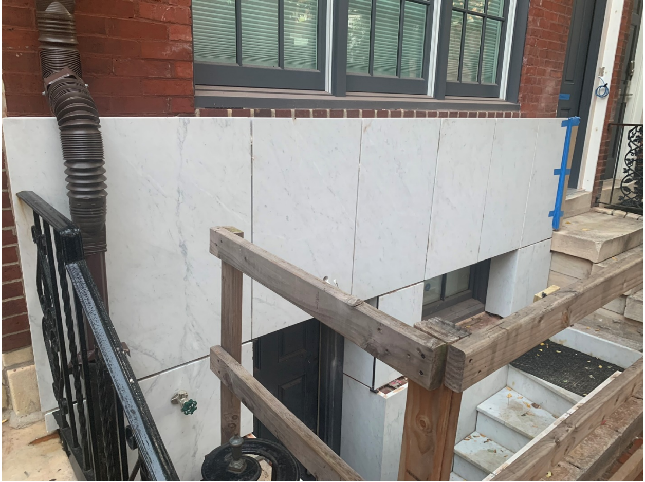
Figure 4. Marble veneer during installation.
