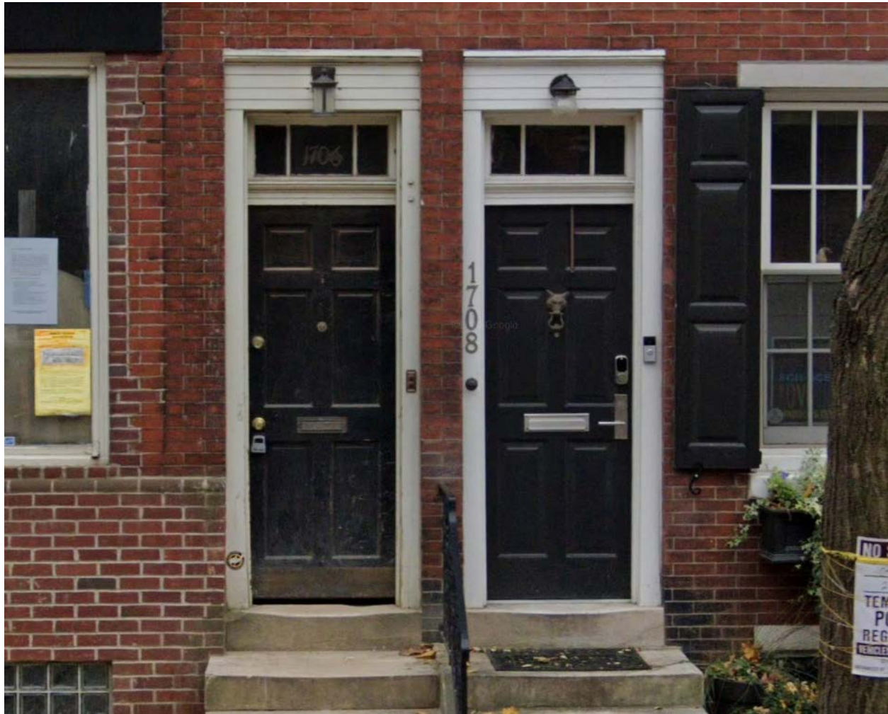
Figure 1. Matching entrances at 1706 (left) and 1708 Delancey Place prior to removal of door frame at 1706 Delancey Place.
