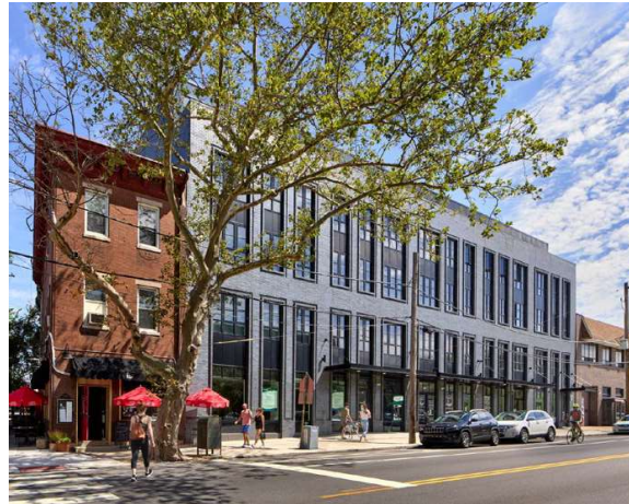
2333 FAIRMOUNT AVENUE Completed 2019
