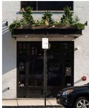
ENTRY CANOPY STEEL CHANNEL FRAME *PHOTO OF 1720 FAIRMOUNT AVE
