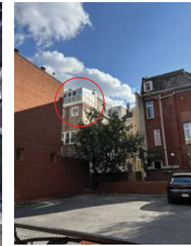
1133 SPRUCE ST. REAR ADDITION
