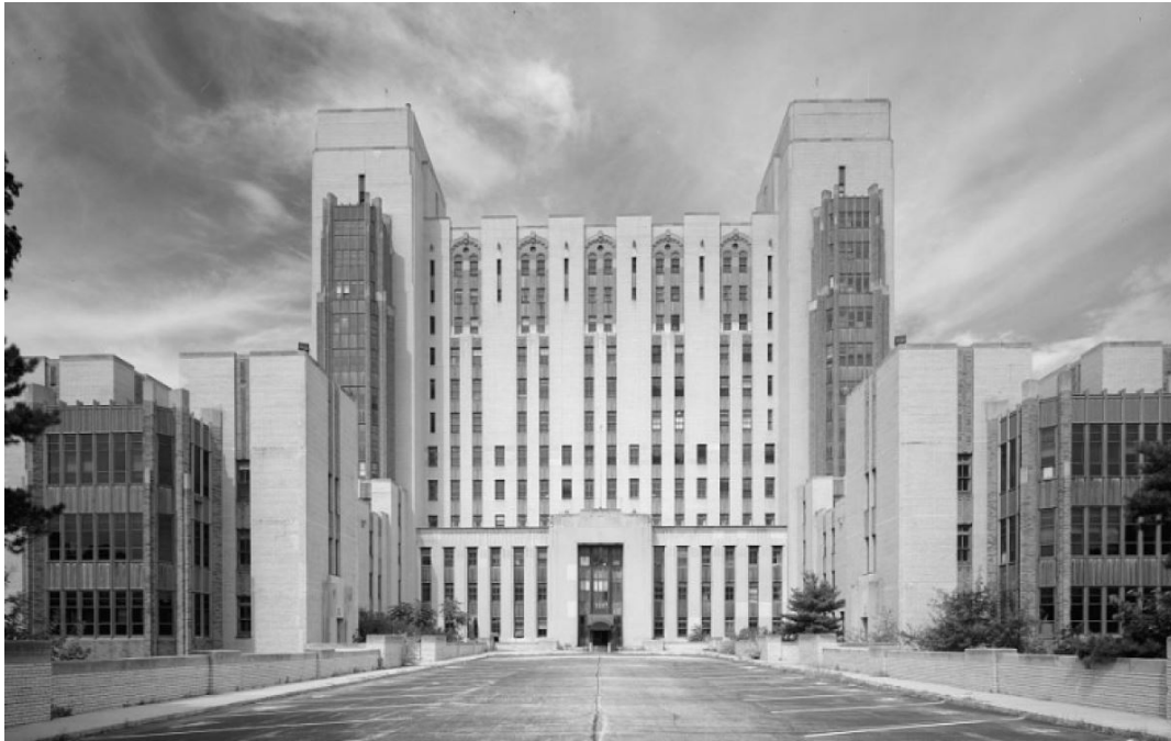
Figure 19: US Naval Hospital, Pattison Avenue between South Broad Street and 20th Street, Karcher & Smith, 1929, demolished 2001. Source: Library of Congress
