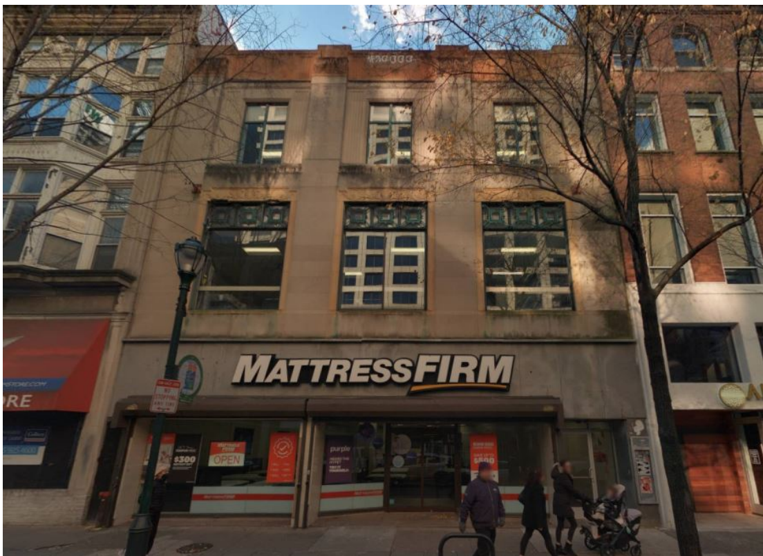
Figure 14: Peck and Peck Store building, 1722-24 Chestnut Street, 1929, Silverman and Levy. Source: Cyclomedia
