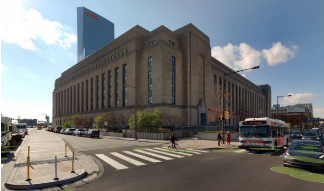
Figure 20: US Post Office building, 2970 Market Street, 1931-35. Source: Cyclomedia
