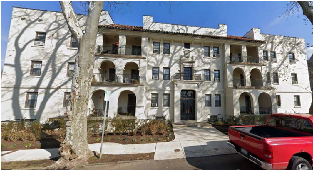
Figure 12: The Hardie apartment building by H.G. McMurtrie, Bala Cynwyd, PA, 1928 25
