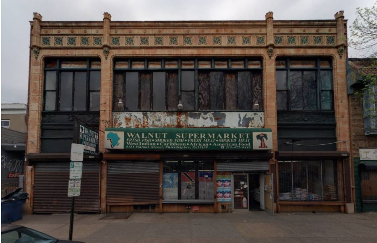
Figure 2. Front façade of 5131-37 Walnut Street looking north, December 2022. Source: Cyclomedia.
