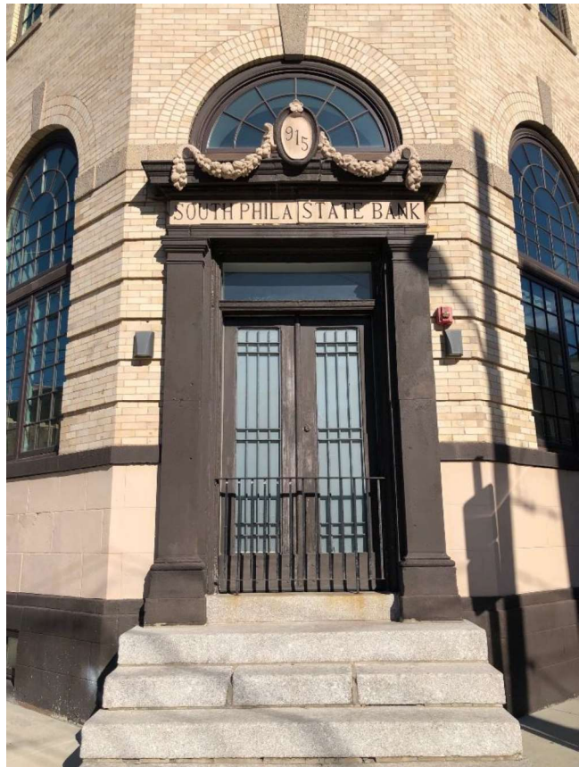
Figure 5: Former main entrance at 11th Street and Montrose Street.
