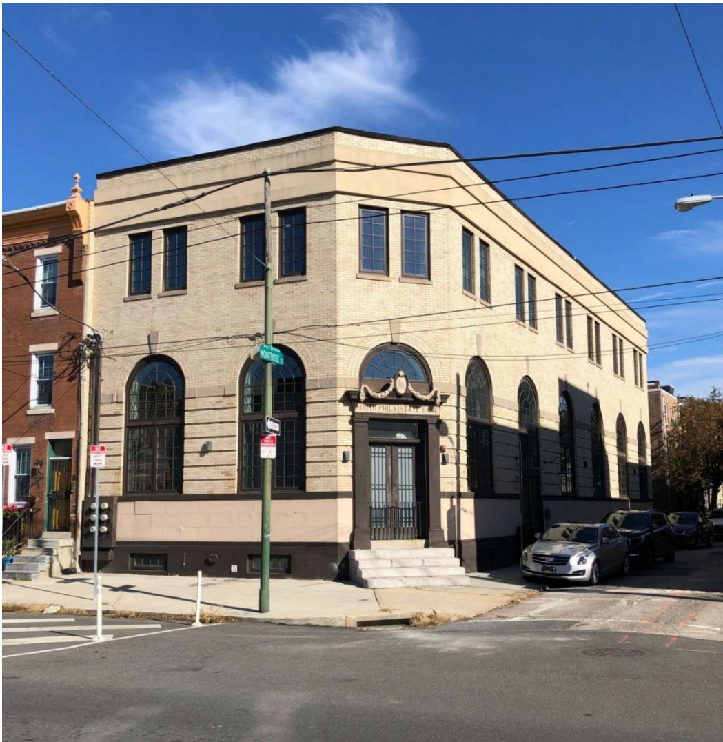
Figure 10: View of building from S. 11 th Street.
