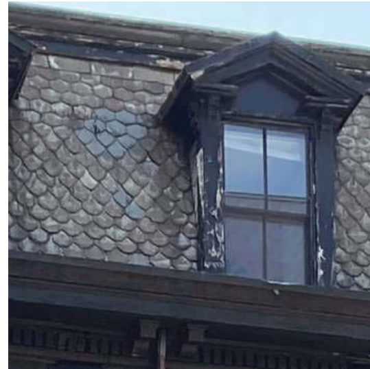
6 Existing Slate Shingles to be Restored
