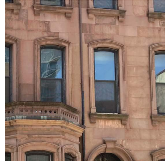
7 Existing Masonry to be Restored
