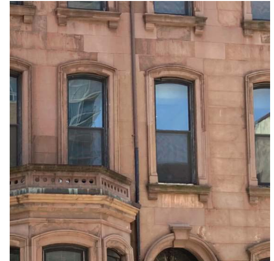
8 Existing Masonry to be Restored
