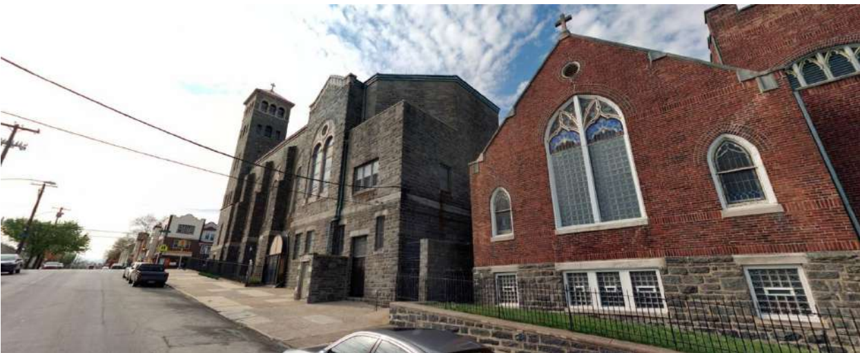
South (side) elevation along Callowhill Street with view of the Protestant church in the foreground referenced throughout the nomination.
