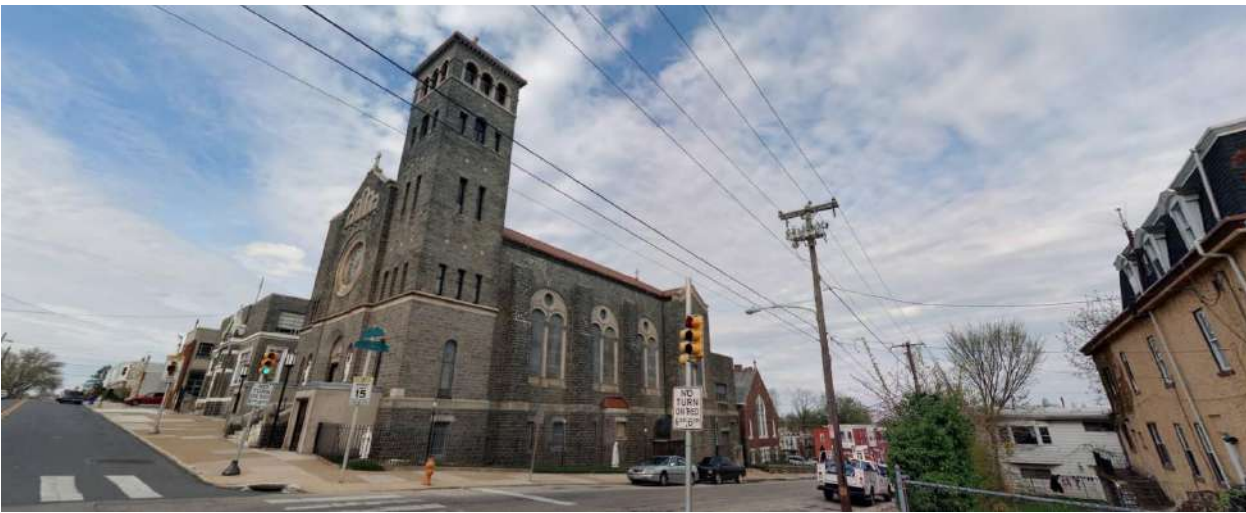
South (side) elevation along Callowhill Street.
