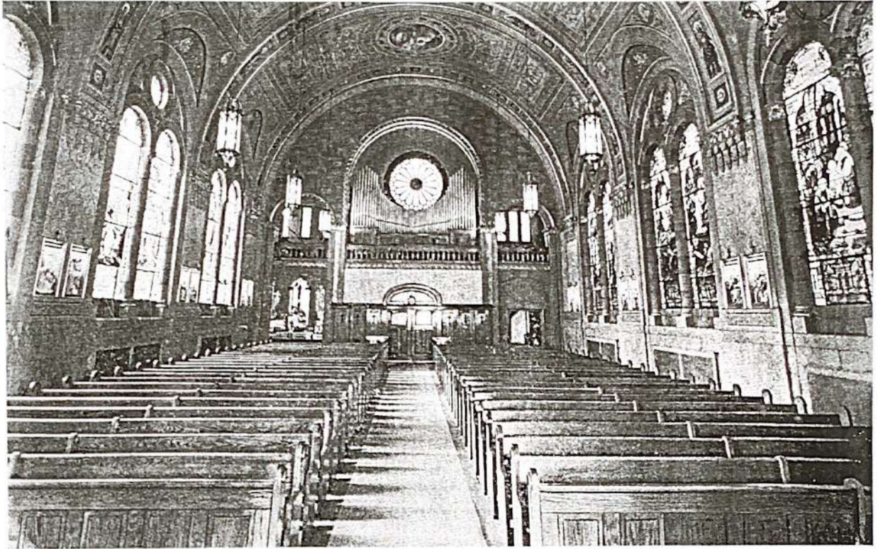
INTERIOR — GENERAL REAR VIEW
