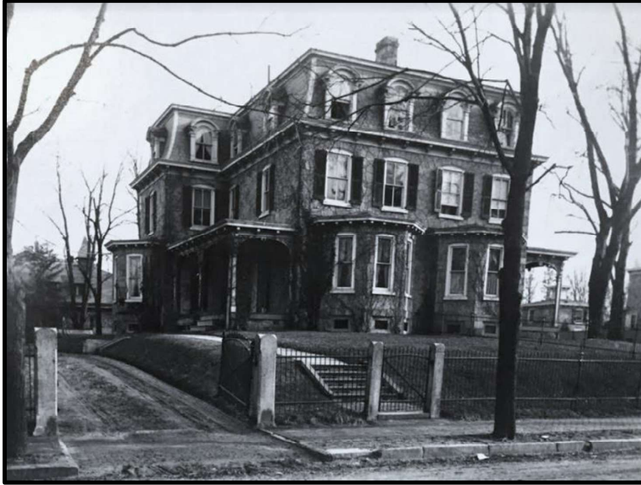
Figure 36. The Rev. George Bringhurst House at 524 Locust Avenue, which is one side of a Second Empire style twin. Source: Wyck House & Garden.
