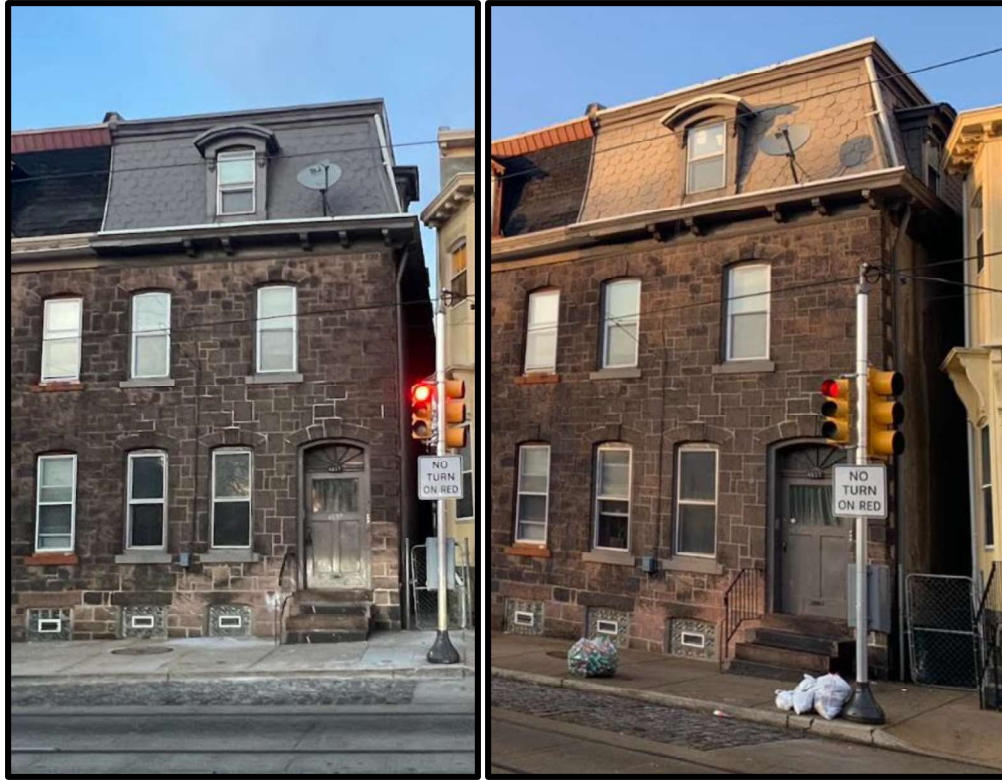
Figure 3a. and 3b. The primary elevation (southwest) elevation of 4837 Germantown Ave. Source: Keeping Society of Philadelphia, 2022.
