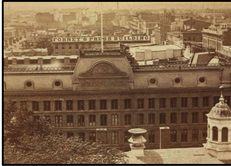
Figure 15. Public Ledger Building, Philadelphia, Pennsylvania, ca. 1867. Source: The Library Company of Philadelphia.
