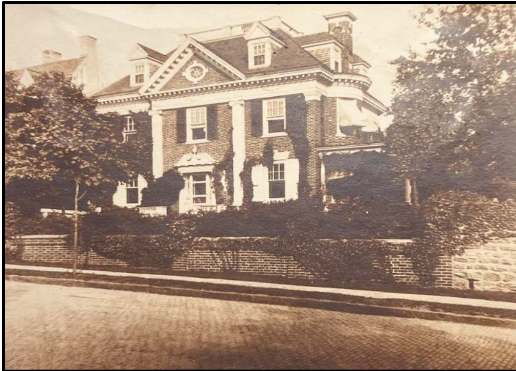
Figure 14. The northwest (primary) elevation of “Cranford” in 1908. Source: Fire Insurance Survey No. 15940, 3 August 1908.
