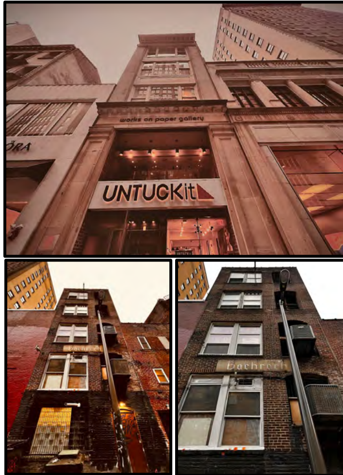
Figure 5. Top: Looking upward at the details within the primary (south) elevation. Figure 6. Bottom left: The rear (north) elevation of the subject property. Figure 7. Right: The rear (north) elevation of the subject property. Source: Oscar Beisert, 2022.
