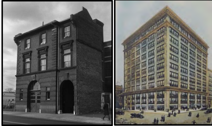
Figure 32. Left: Fire Engine Co. No. 47 at 3035-37 Gray’s Ferry Avenue designed by Charles E. Oeschlager. Source: PhillyHistory.org. Figure 33. Right: A Beautifully Detailed, Original Plan of the Sales and Service Building for Gomery-Schwarz Co. designed by Oeschlager, published in the American Architect and Building News on 5 June 1918. Source: St. Croix Architecture.
