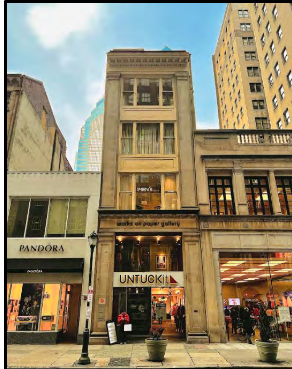
Figure 1. The primary (south) elevation of the subject property. Source: Oscar Beisert, 2022.
