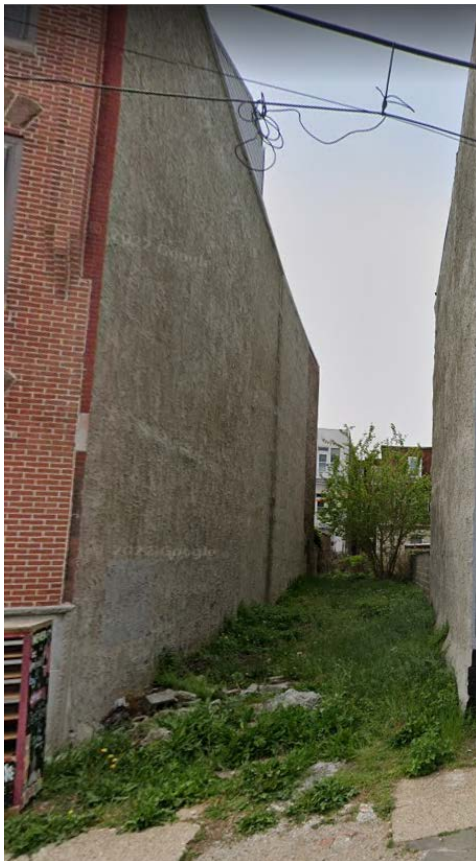
Figure 7: North Elevation. Source: Google Earth
